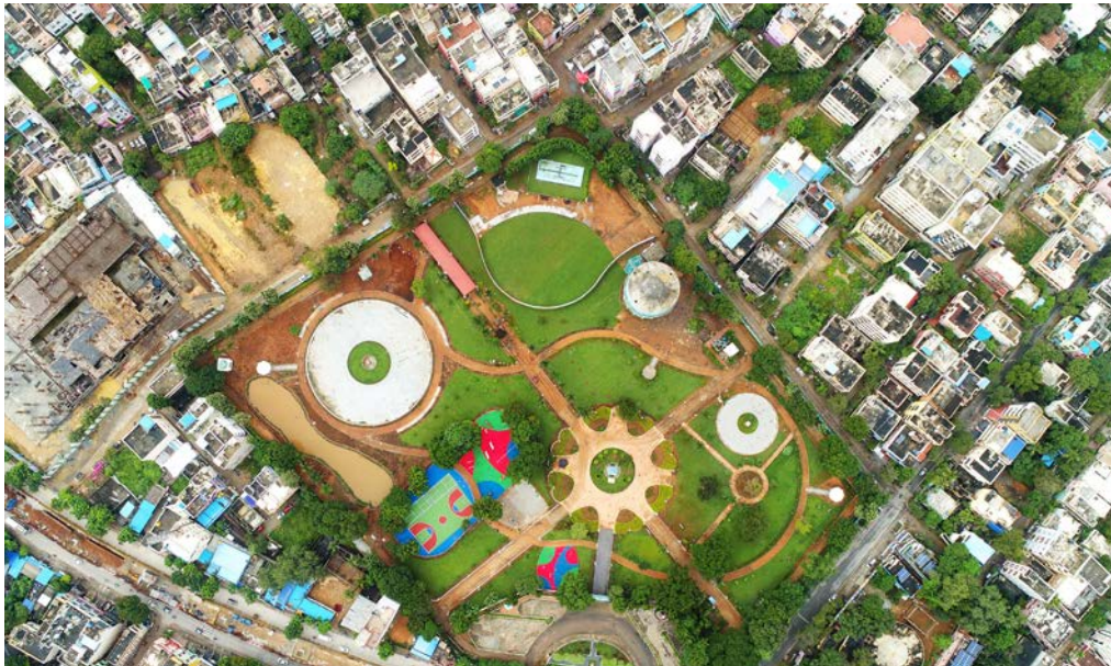
A refurbished park in Tirupati
