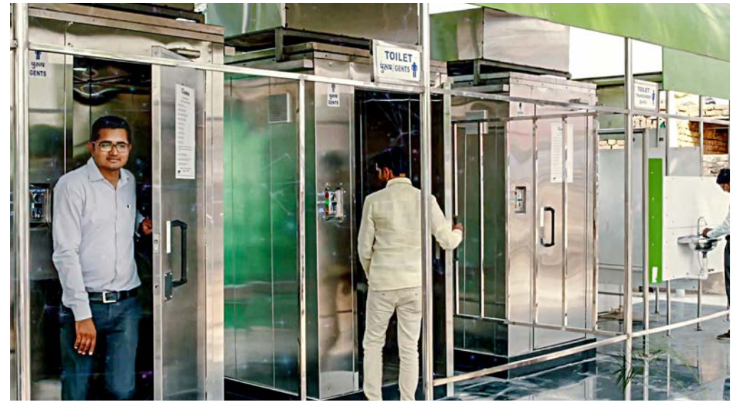
Citizens using self-cleaning smart public toilet in Agra
