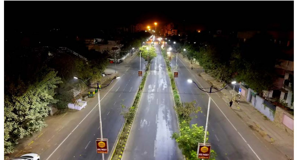
Smart LED streetlights in Ahmedabad
