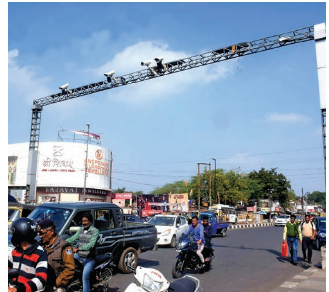
Bhopal Intelligent Traffic Management System (ITMS)
