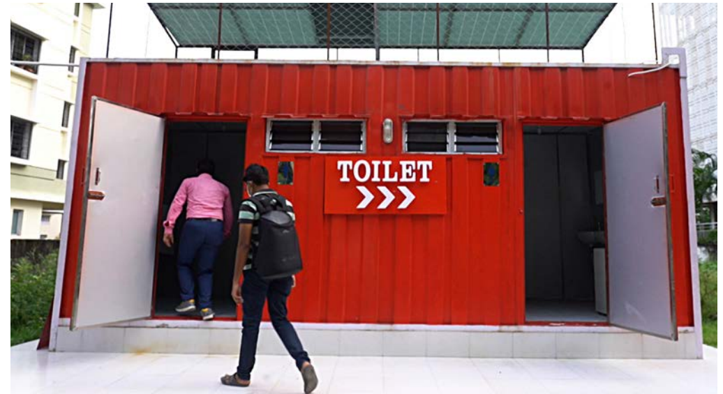
Containerised public toilets in New Town Kolkata
