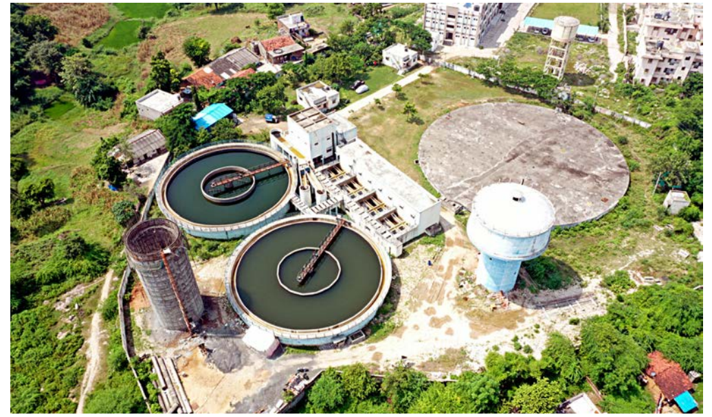
Water supply project in Dahod
