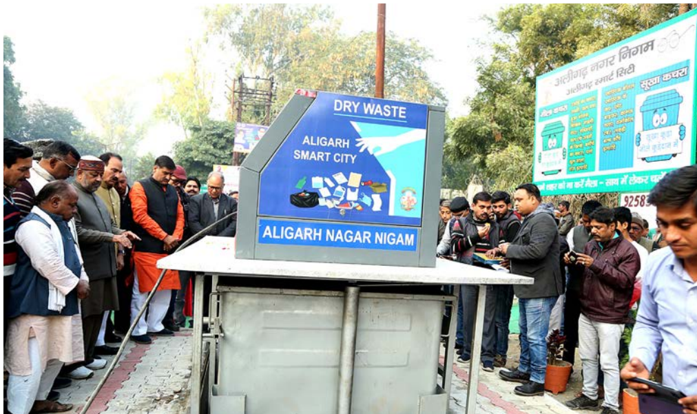
Underground dust bins installed by Aligarh are an efficient and accessible way of collecting waste and recycling materials
