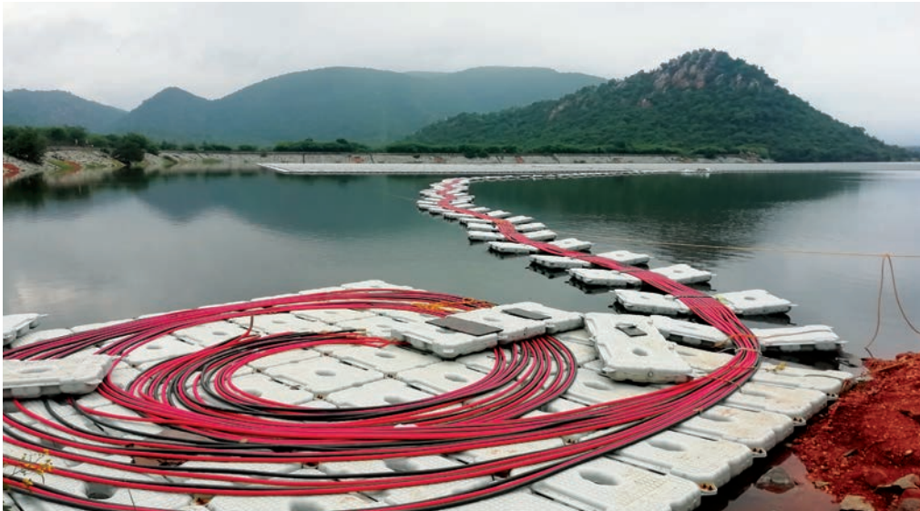
Floating solar project installed in Tirupati
