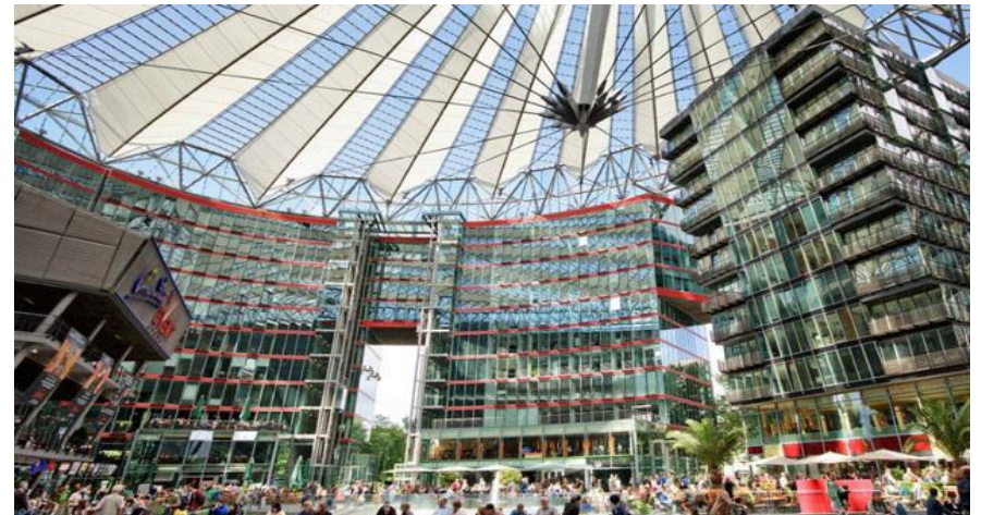
Potsdamer Platz – The Largest inner city Reconstruction in Europe. Renzo Piano designed DaimlerChrysler District and features architecture by renown practices such as Rafael Moneo, Mies van der Rohe & Richard Rogers.
