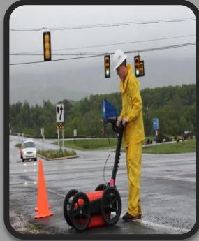
Road & Highway Inspection
