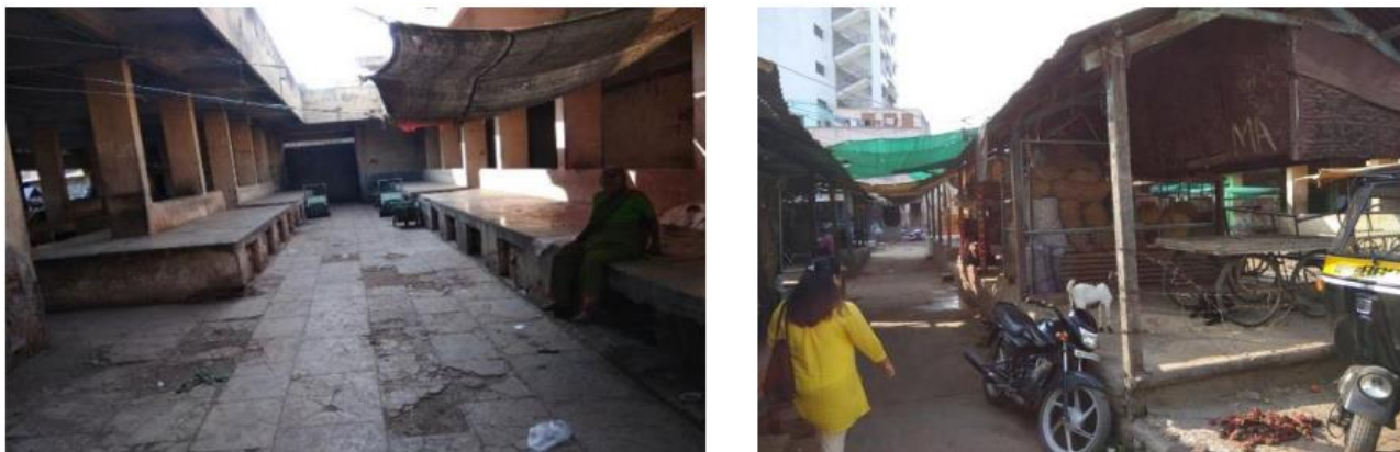
Figure 1-4 Unmanaged Flooring and Vacant Ottas
