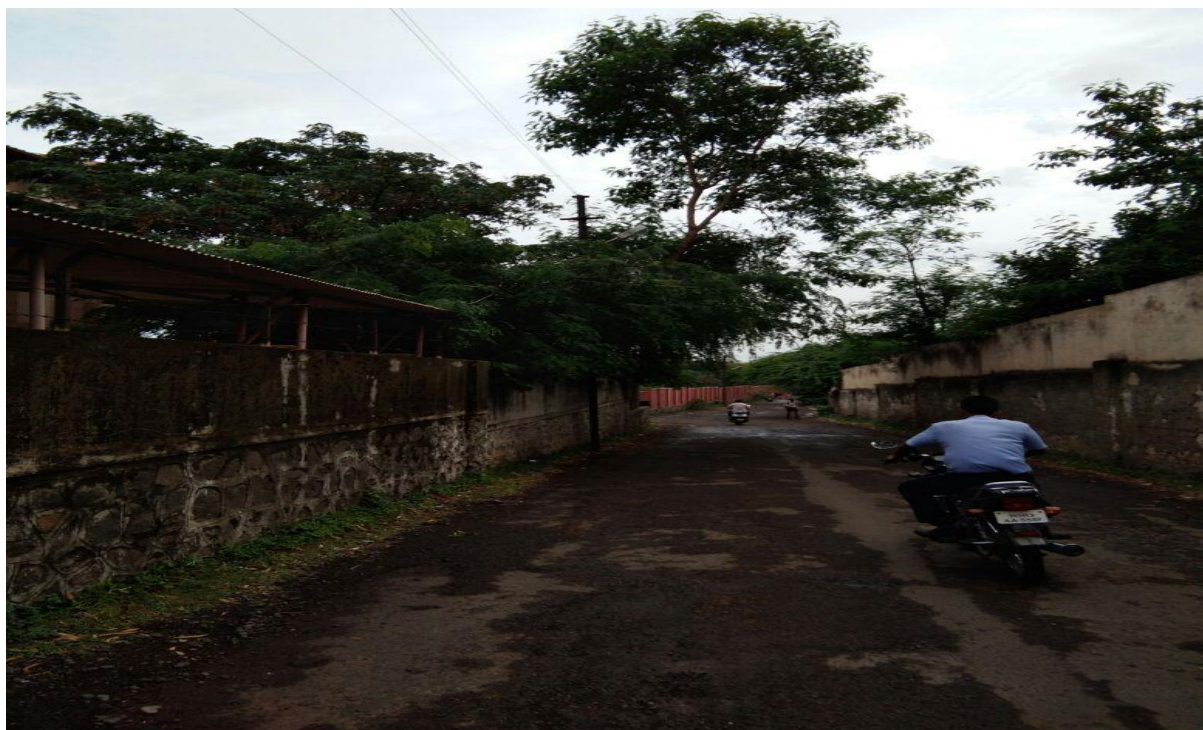
Img 8 : Surface Coat Damaged.
