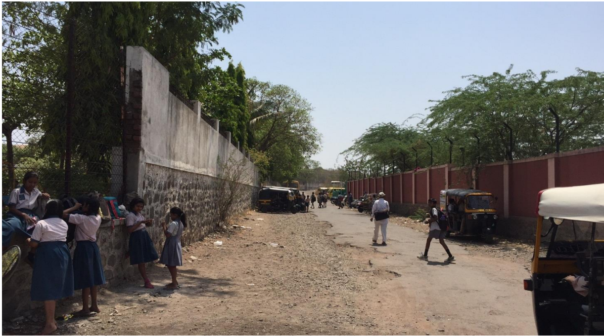
Img 2 : Tar Finish is present only on Partial Surface
