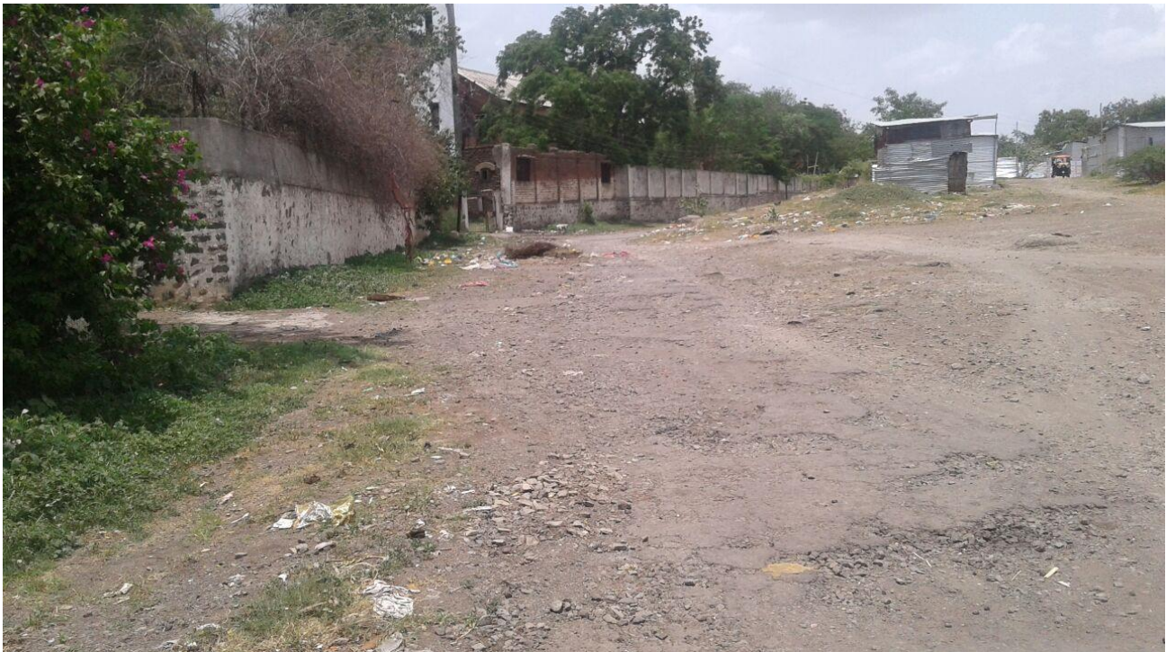
Img 3 : Damaged Tar Surface
