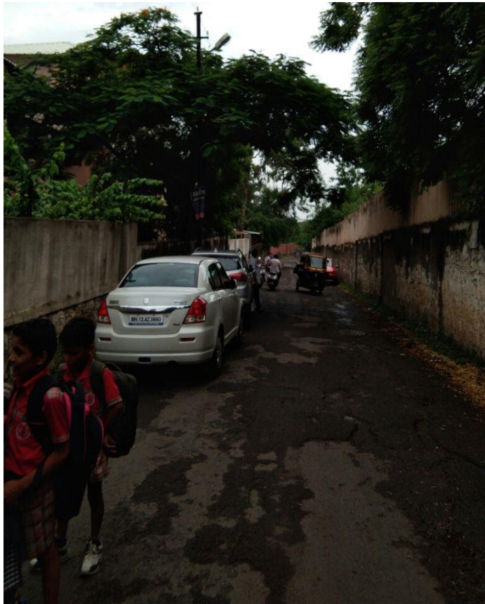
Img 9 : Tar Surface not in good condition
