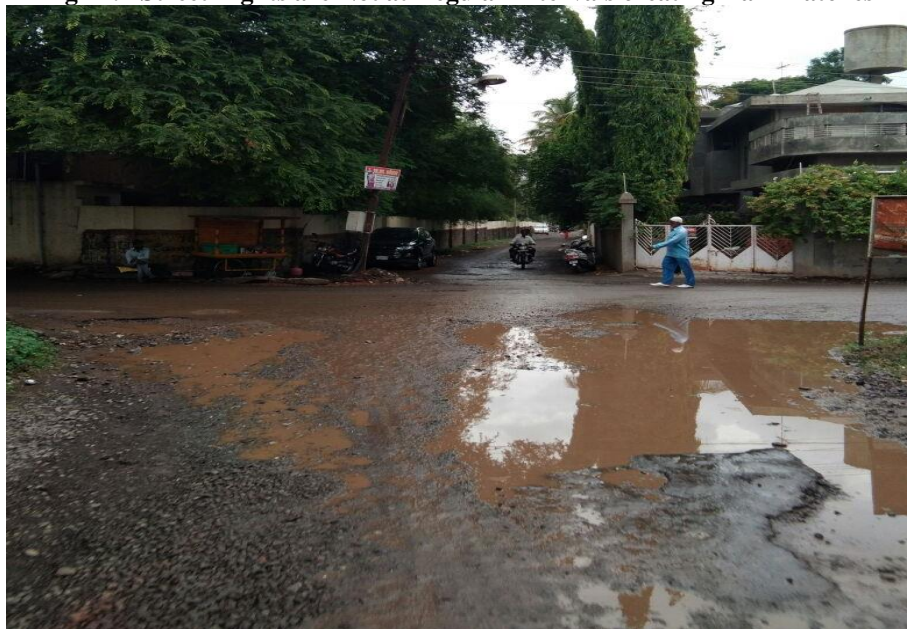
Img 12 : Pot Holes at the Junction , Near Cementary
