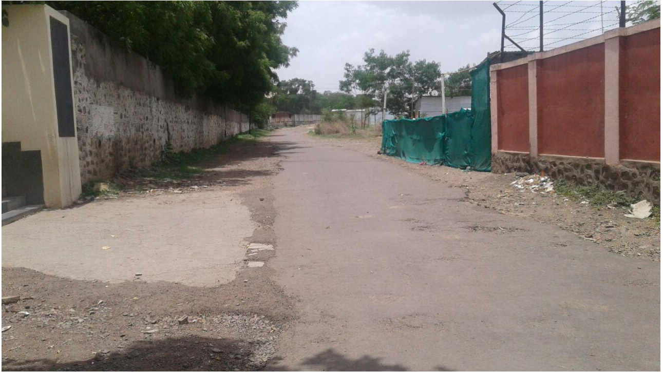
Img 6 : Damaged Tar Surface due to Storm water from Weep Holes of Haribhai School Ground.
