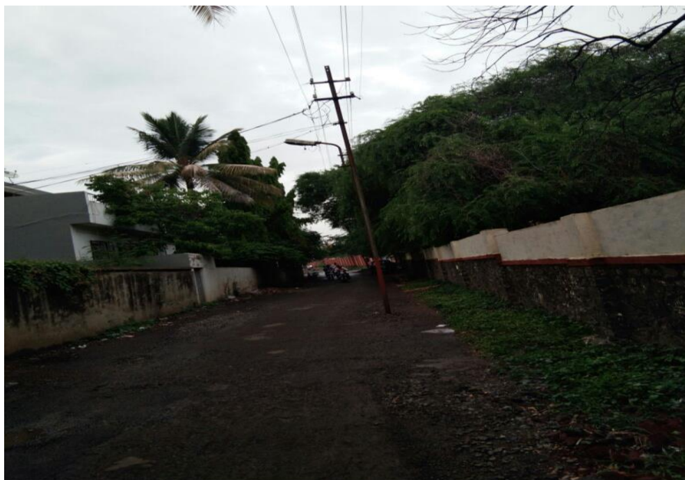
I mg: 15 - Tar Surface in Bad Condition
