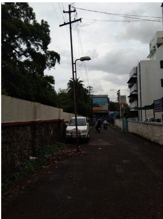
Img: 14 - Compound wall on both Sides
