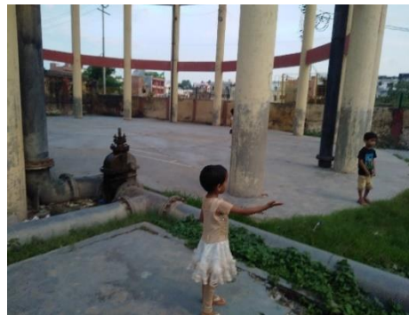
Existing Overhead Tank
