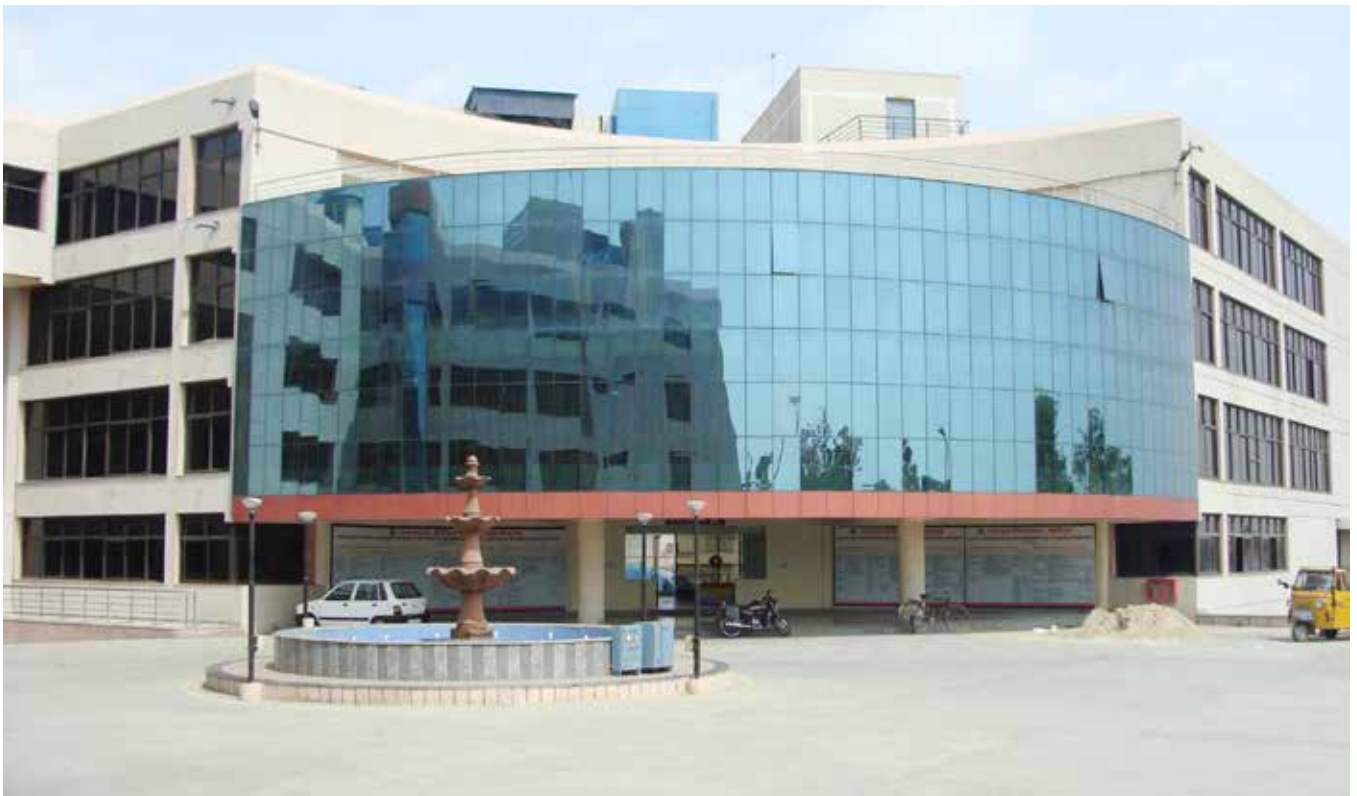
KOTA MUNICIPAL CORPORATION BUILDING
