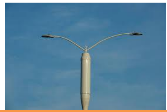
iPoles integrated with Command and Control Center
