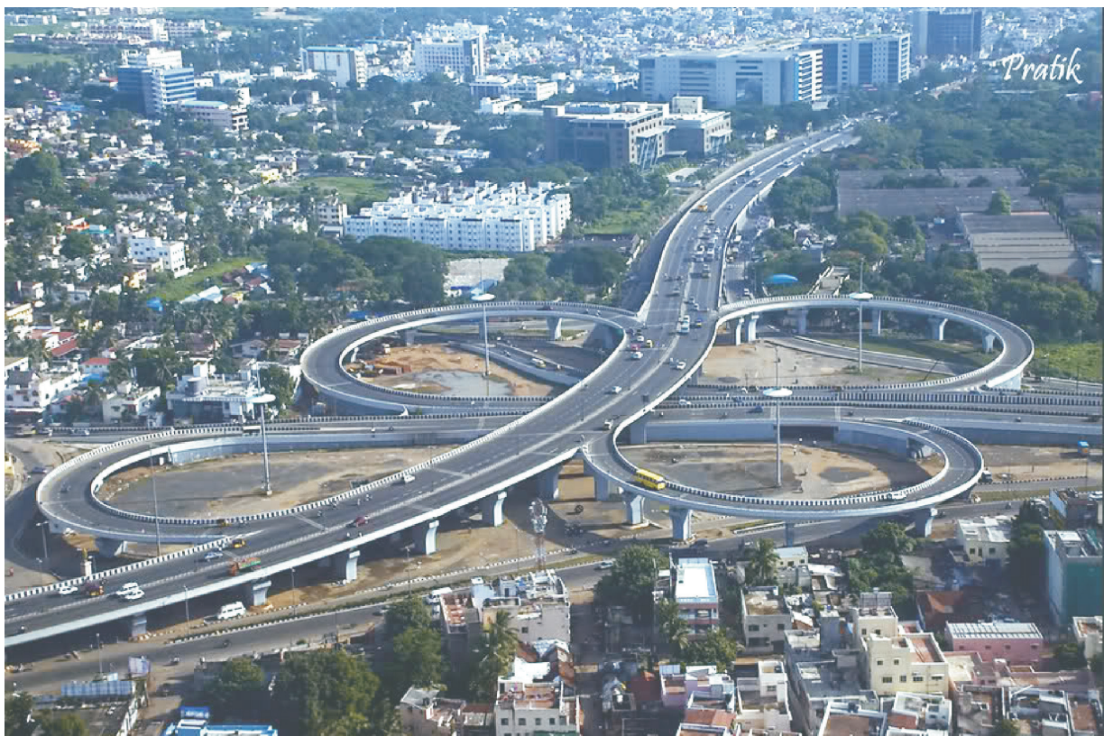
Photo 7.1: Kathipara cloverleaf interchange constructed in place of a roundabout
