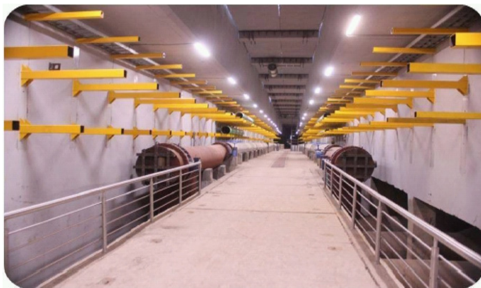
Figure 12 – Utility Tunnel, showing support brackets [Source: Nilesh Puery, b-2]
