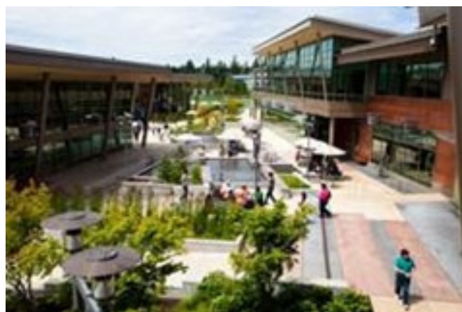
Figure 5 – Microsoft Headquarters Pilot Building
