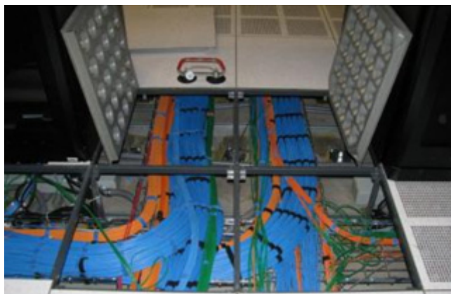
Figure 10 – Under floor cable runs
