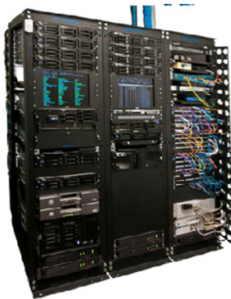
Figure 12 – Rack mounted servers
