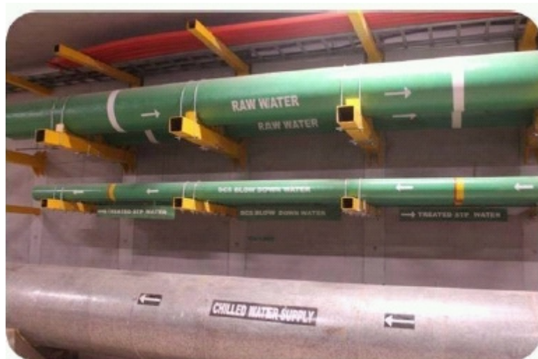
Figure 13 – Utility Tunnel, showing waste and water pipes [Source: Nilesh Puery, b-2]
