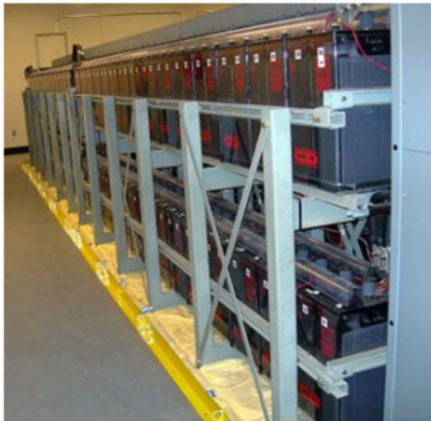
Figure 11 – Bank of batteries
