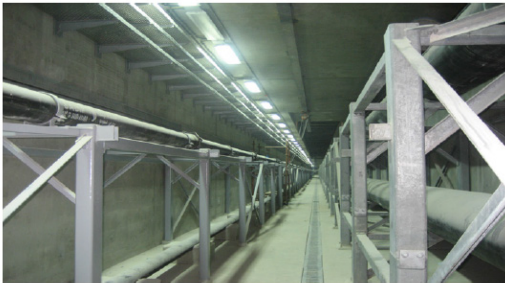
Figure 4 – Example of utility tunnel [Source: Abu Dhabi Utility Corridors Design Manual, b- 1]
