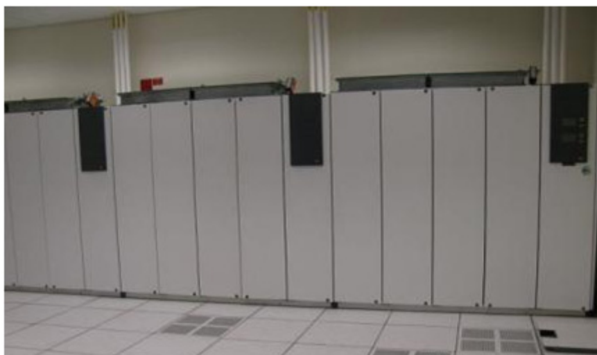
Figure 13 – Air conditioning equipment
