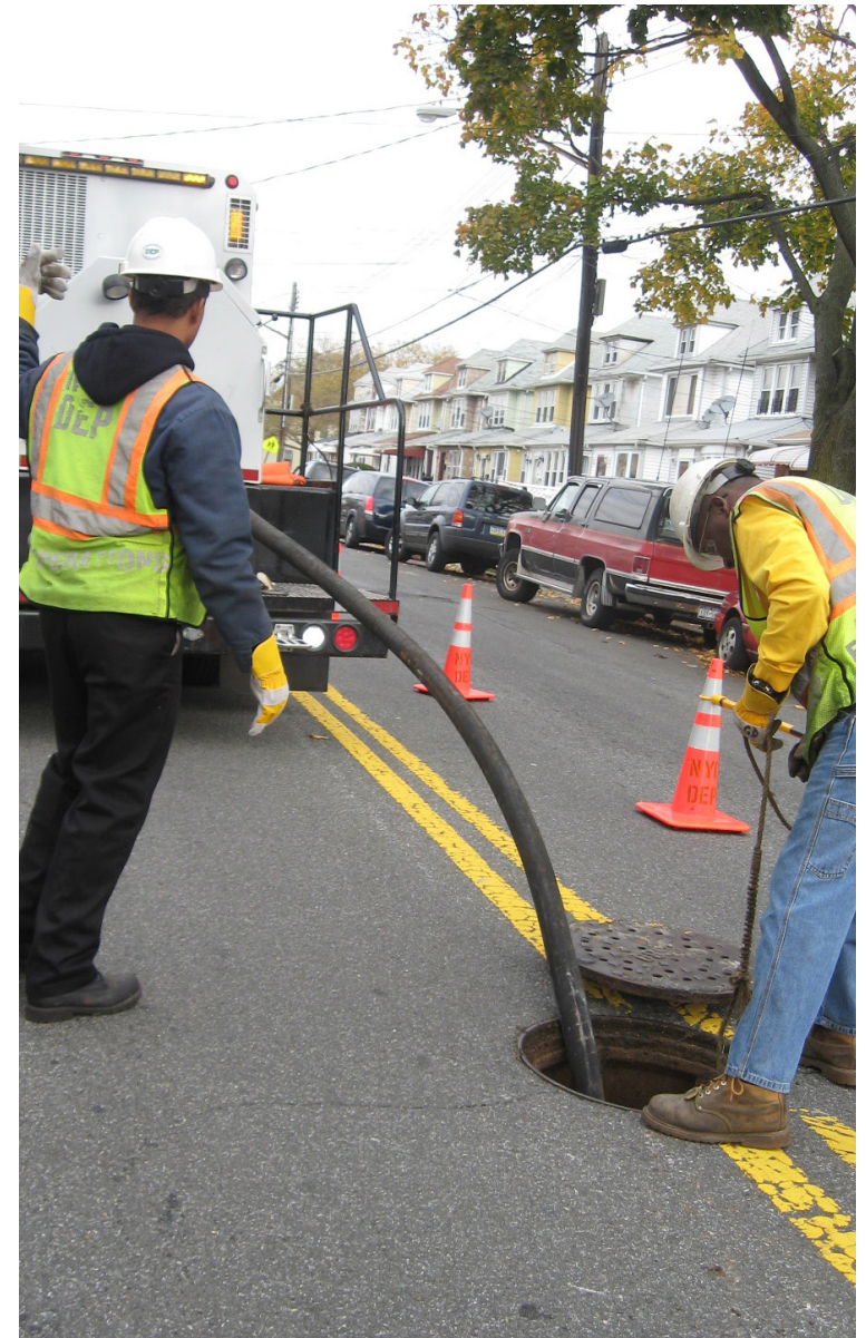
Sewer Flushing
