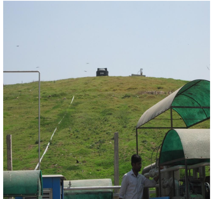
Capping and gas recovery
