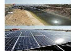
Solar panels generation 1. Green zone along the canal
