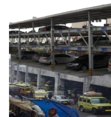
Retrofitting and Expansion of 3 MUDA Parking Complexes
