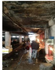
2- Poor drainage network along the corridor of the building
