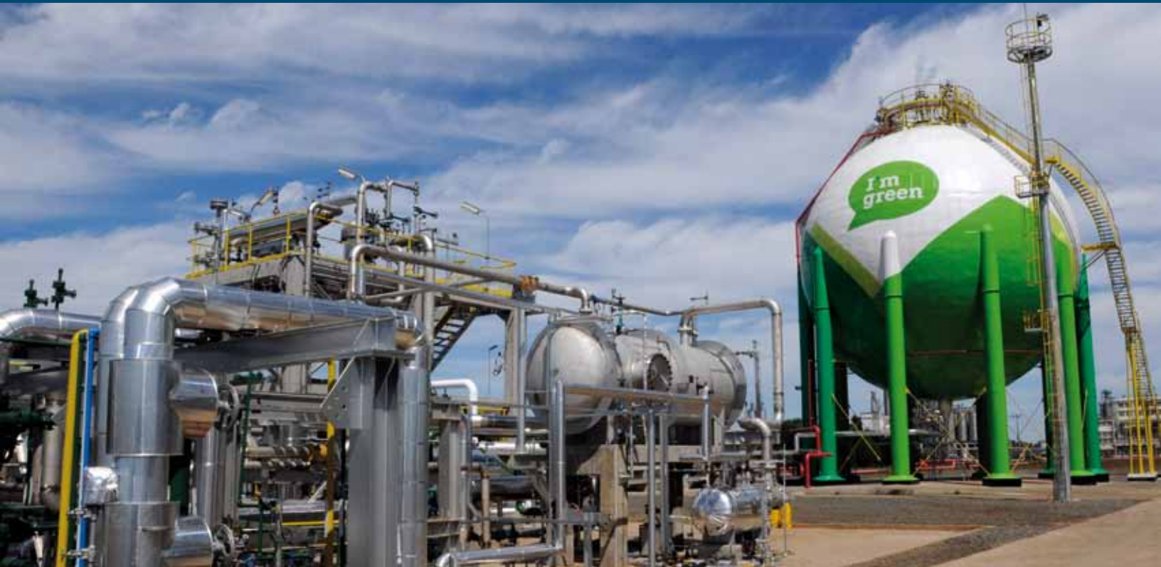
Braskem Ethanol-to-Ethylene Plant, Brazil
