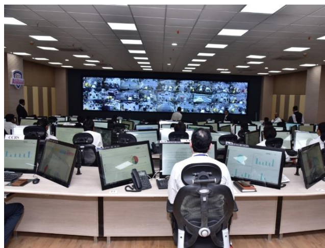
Command Control Centre Video wall
