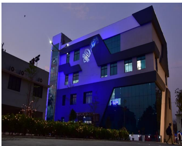
Command Control Centre
