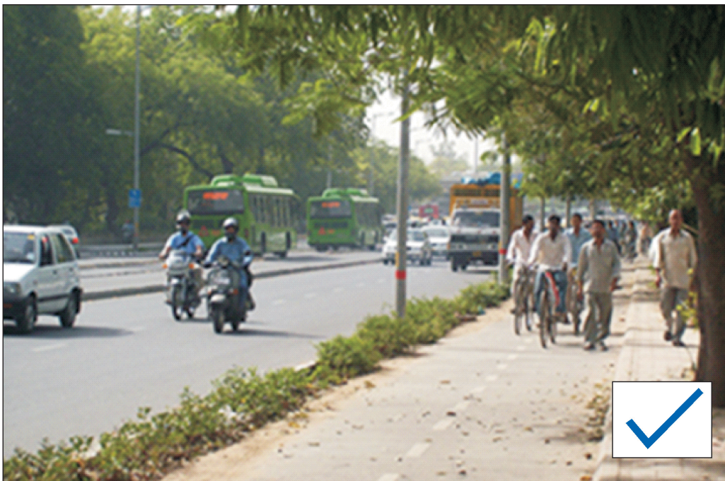
Figure 3.2: Wide, Segregated and Unobstructed cycle track
