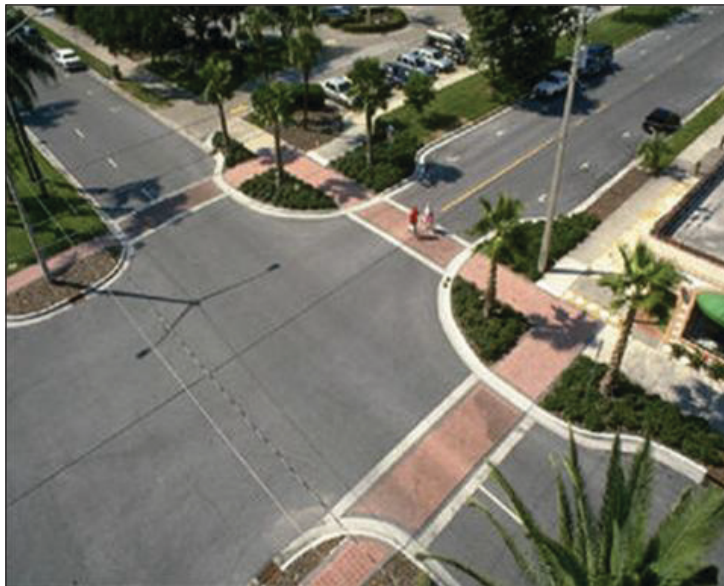
Figure 17.7: Traffic Calming measures at intersection
