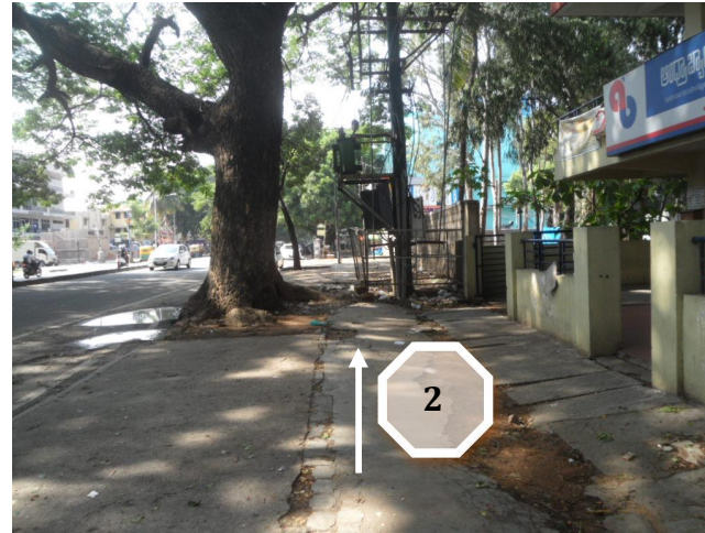
2. Trees and electrical utilities occupying whole of the footpath width resulting in disconnected footpath.
