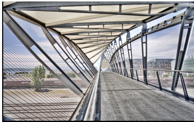
Figure 30b: Example of well-designed pedestrian Bridge, HELIX Pedestrian Bridge, Seattle.
