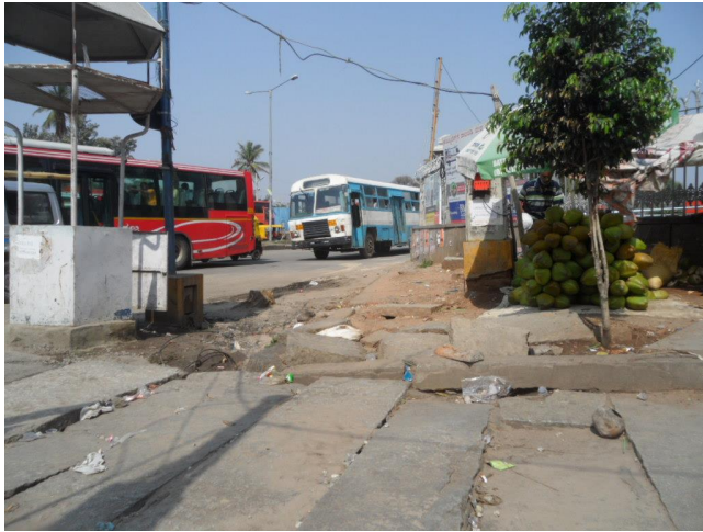
1. No footpath available for pedestrians to walk in the direction of the arrow.
