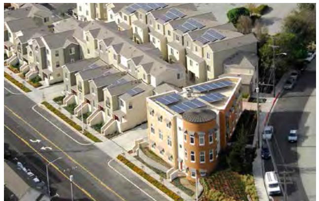
RECOMMENDED - Photo voltaic panels should be included on new developments.
