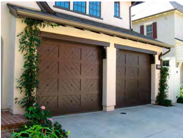
RECOMMENDED - High-quality wood garage doors with decorative wood corbels and header.
