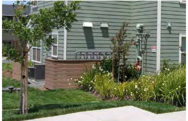
RECOMMENDED - Meters and other utilities should be screened with landscape or low walls when above ground.
