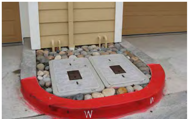
NOT RECOMMENDED - Meters and other utilities located within previously planned landscape areas due to conflicts with plan coordination.
