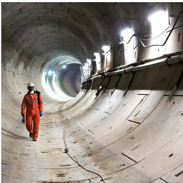
Tunnel inspections near Fisher Street, Holborn. © Crossrail
