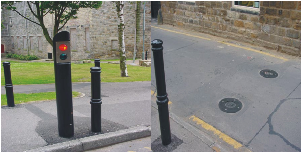
Figure 4.4: Access control & Retractable bollards
