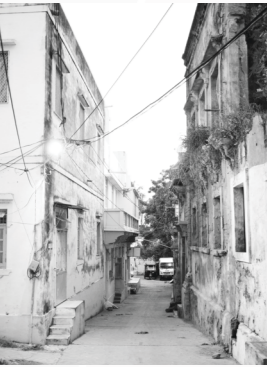
POOR INTERNAL CONNECTIVITY
