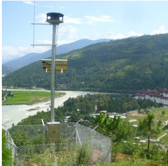
Figure 8: GLOF early warning station
