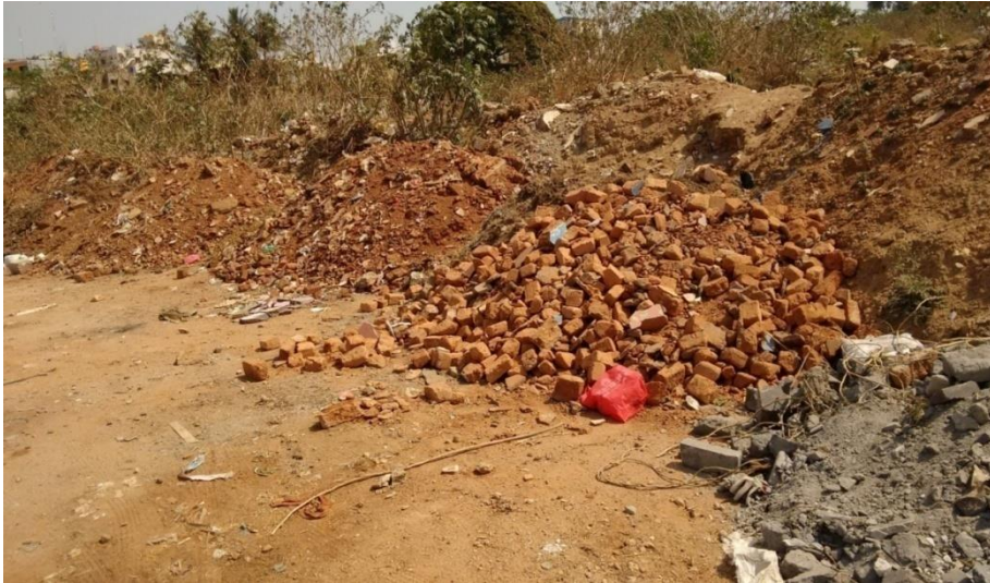
Figure 4: CDW at Mallasandra site
