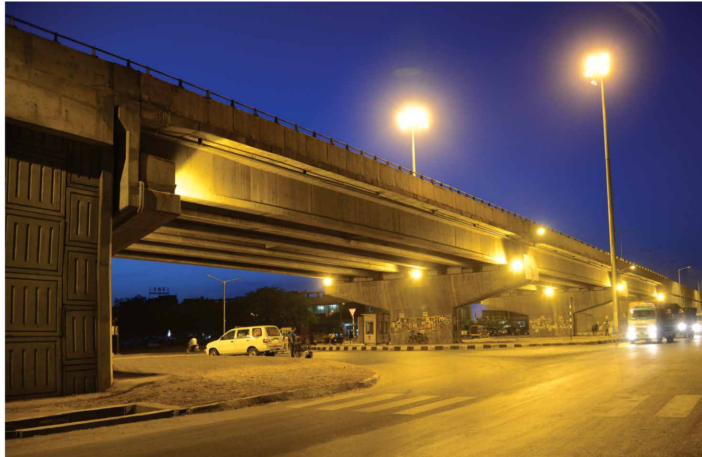
One of the flyovers
