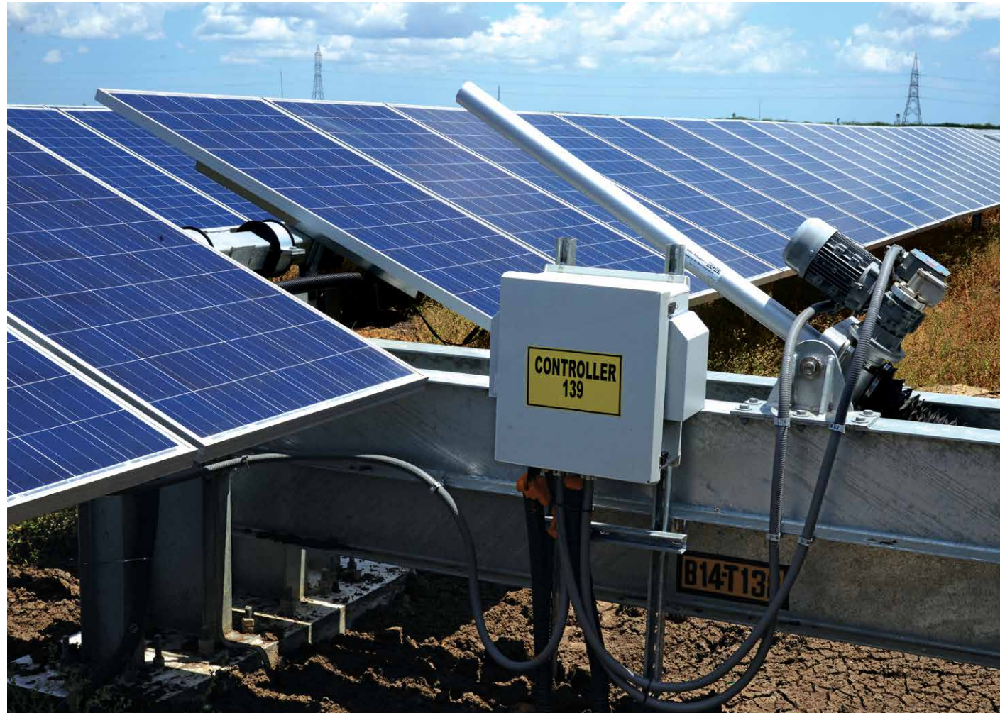
Close-up view of the auto control panel
