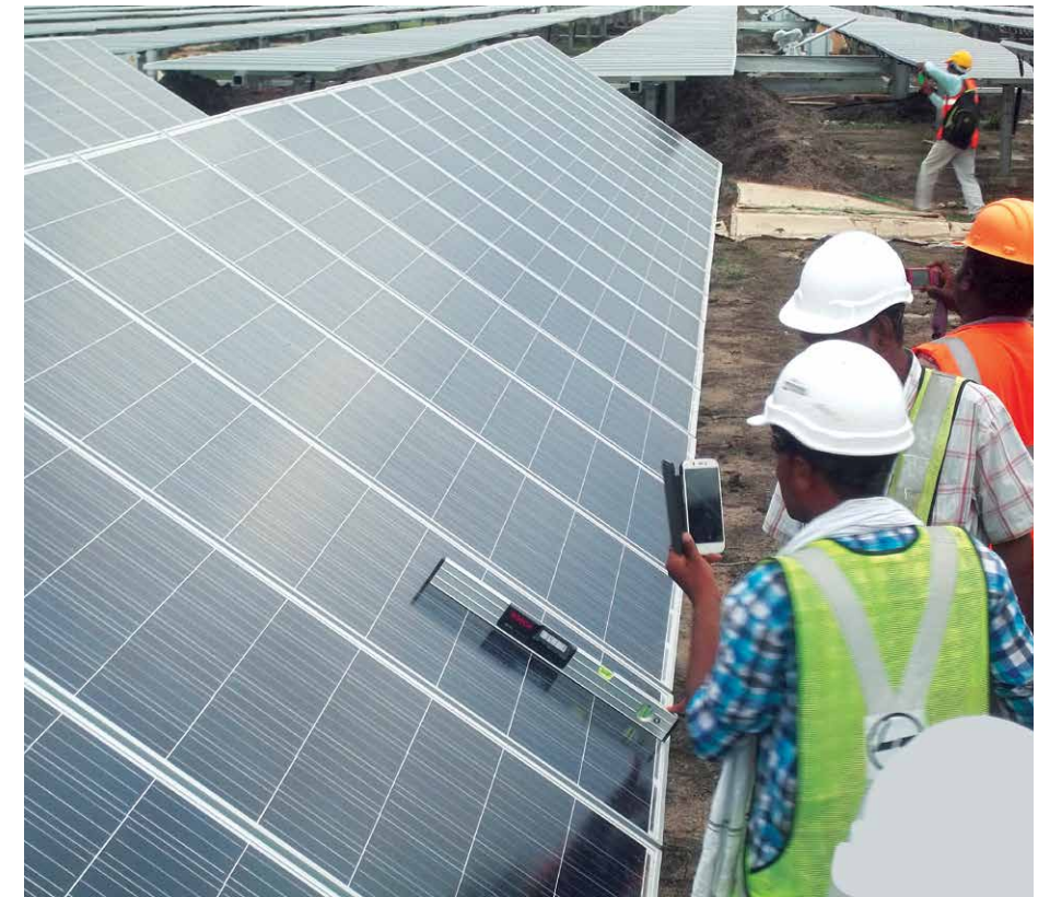
Solar team checking the alignment of the modules
