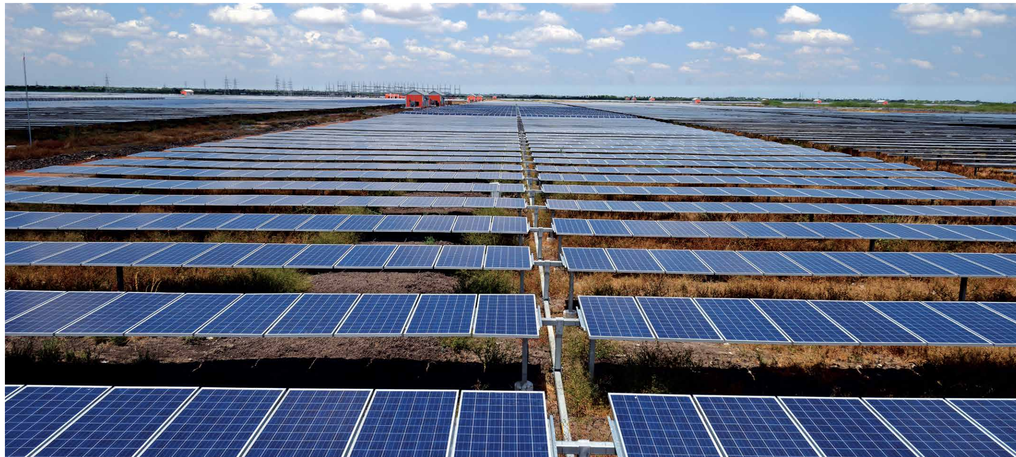
India's largest (60 MWp) tracker based solar plant near Tiruchuli
