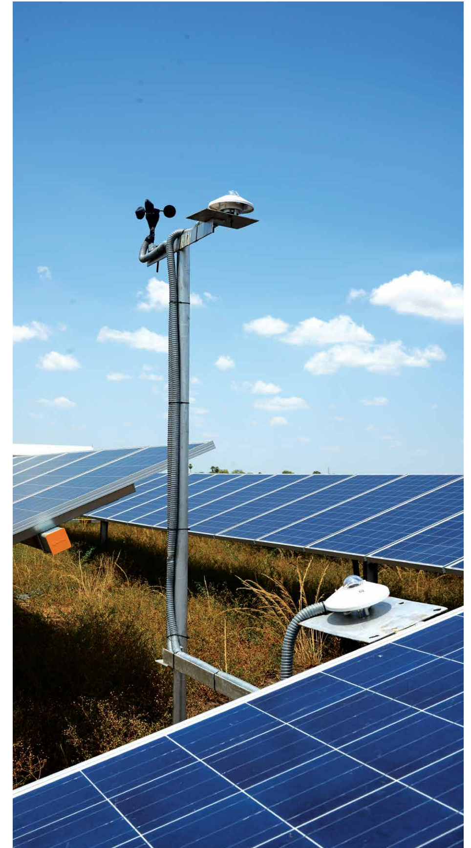
One of the mini weather stations installed across the plant
