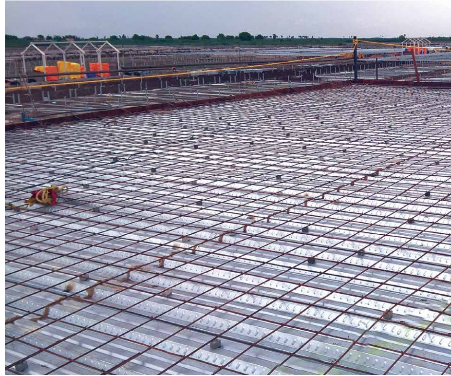
MCR Slab casting
