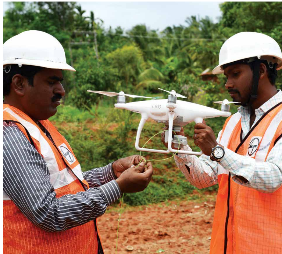
Drone technology deployed to cross over live line
