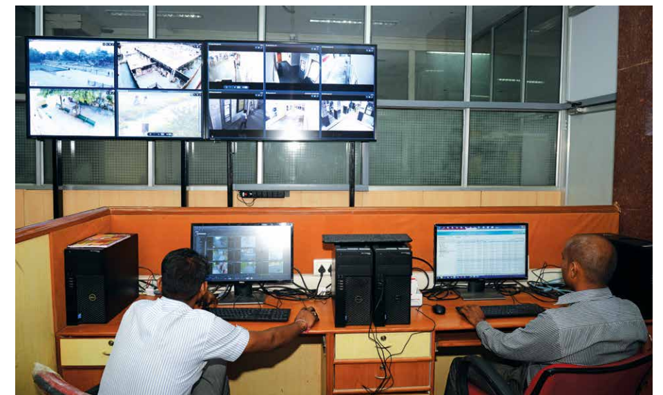
Command and control centre
