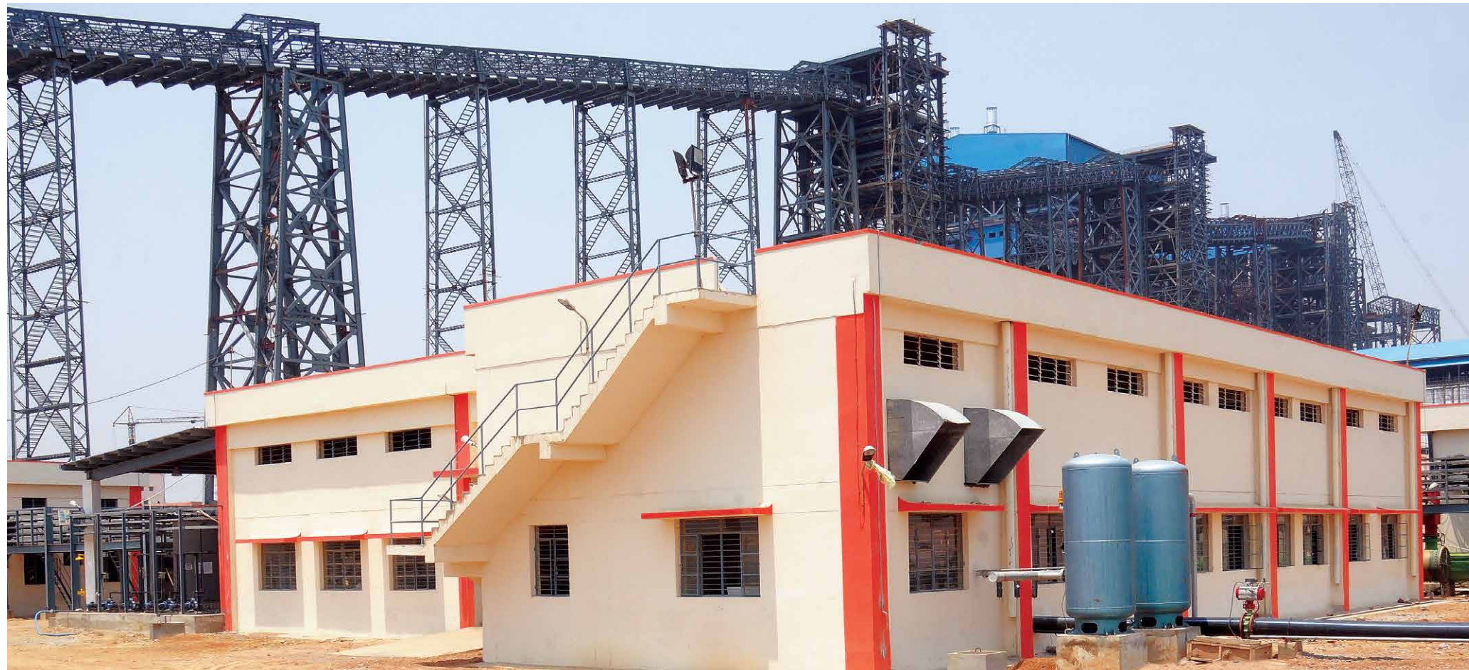
Micro filtration building
