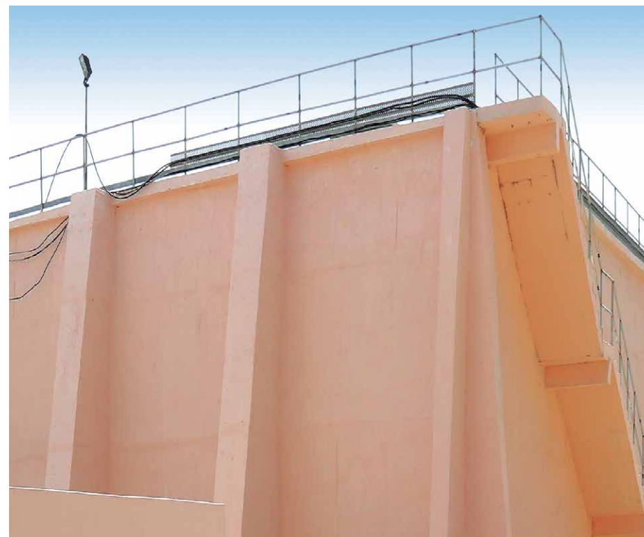
Filter water storage tank
