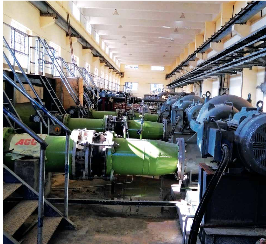
MF Feed pump house
