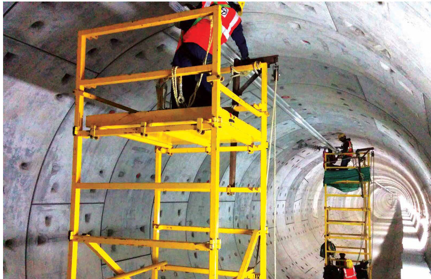
Conductor Rail installation works in progress
