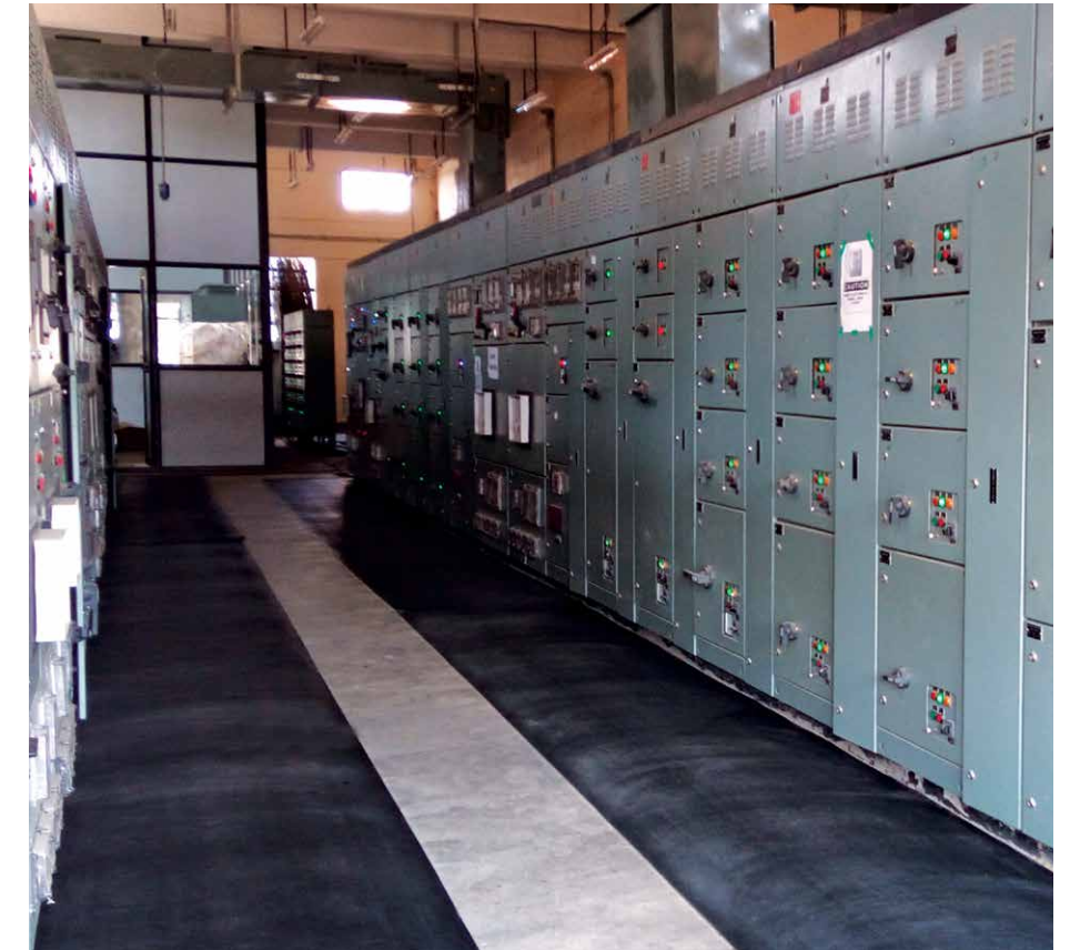
Main control room
