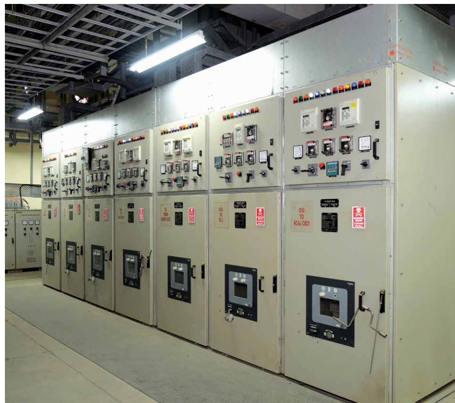
Control panels being installed at one of the stations
