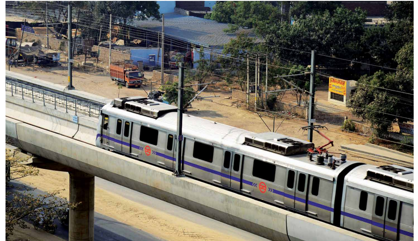
Revenue operation started in Line 6 (Badarpur – YMCA Chauk, 28 tkm) on September 6, 2015
