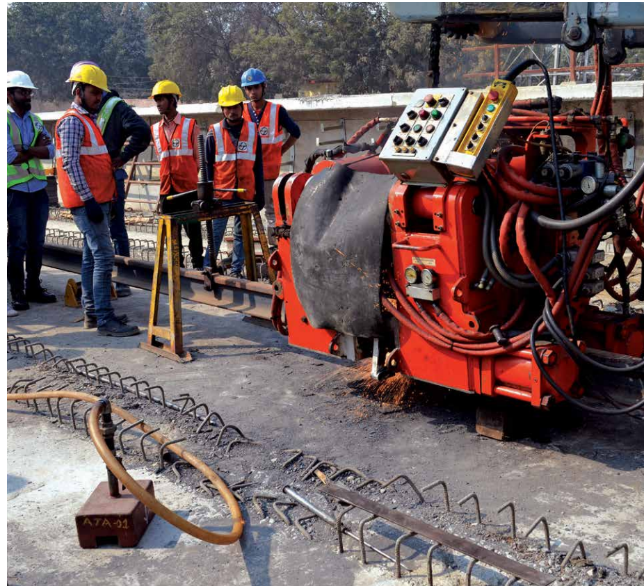
Flash Butt Welding of tracks in progress
