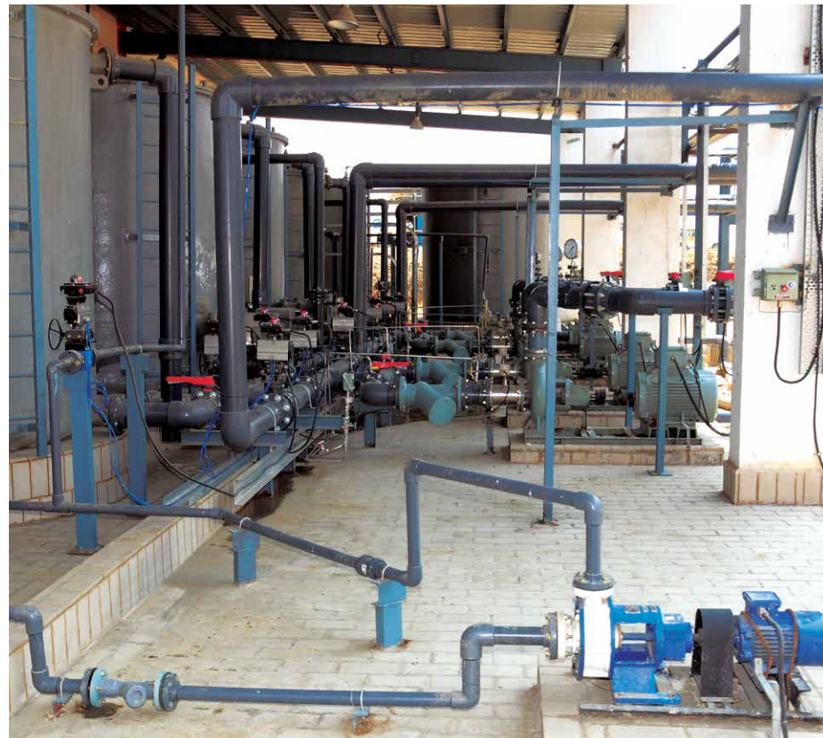
MF Dyke area
