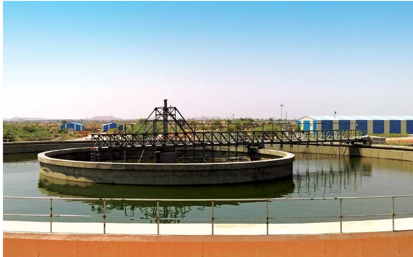
Ash water clarifier
