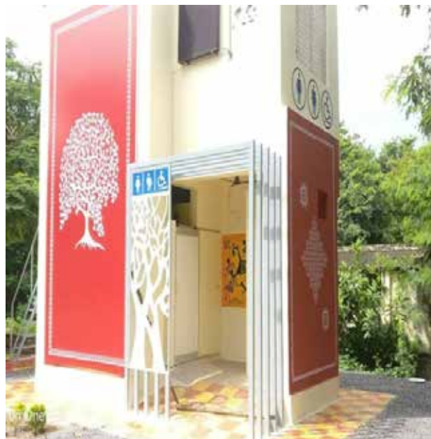
Improved public and school toilets
