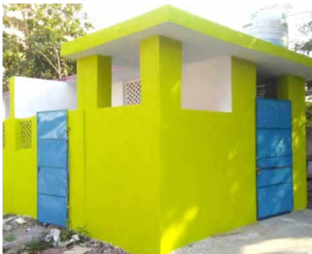
Improved public and school toilets
