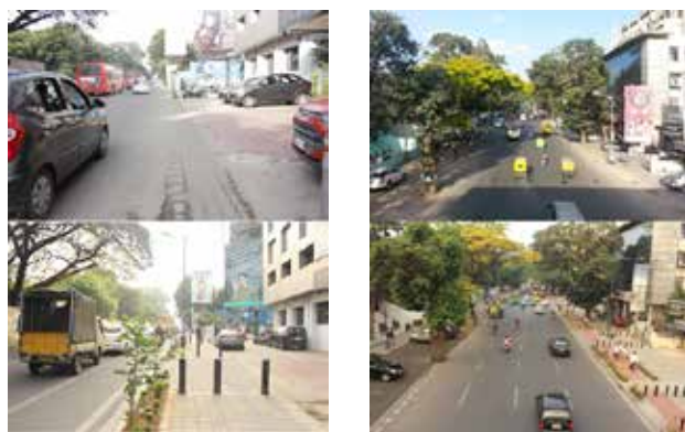
Road Conditions before and after redesigning with the guidelines of tender S.U.R.E
