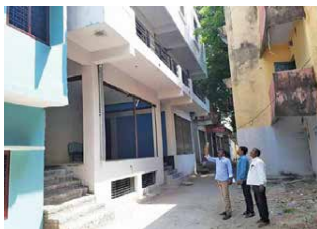
Data collection with the help of mobile application as a part of Survey
