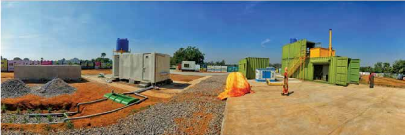
Fecal Sludge Treatment Plant (FSTP) Plant
