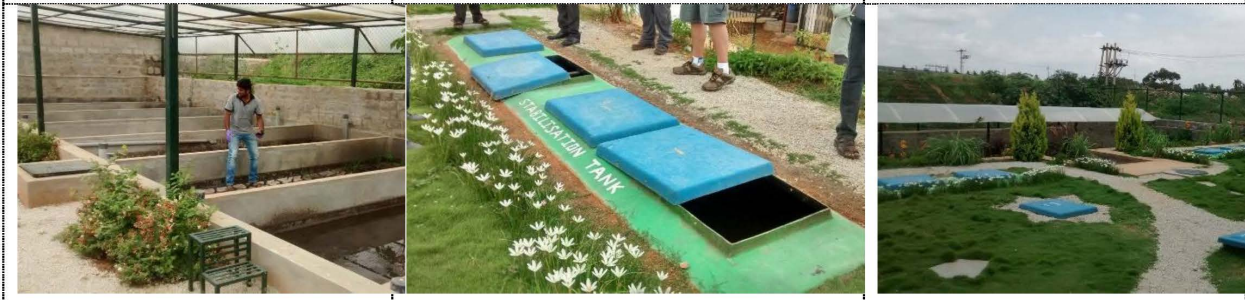
Sludge drying beds Stabilization tank Overview of plant
