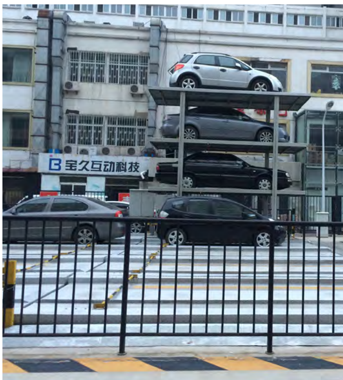
Each lift contains four parking spaces, of which one at ground floor
