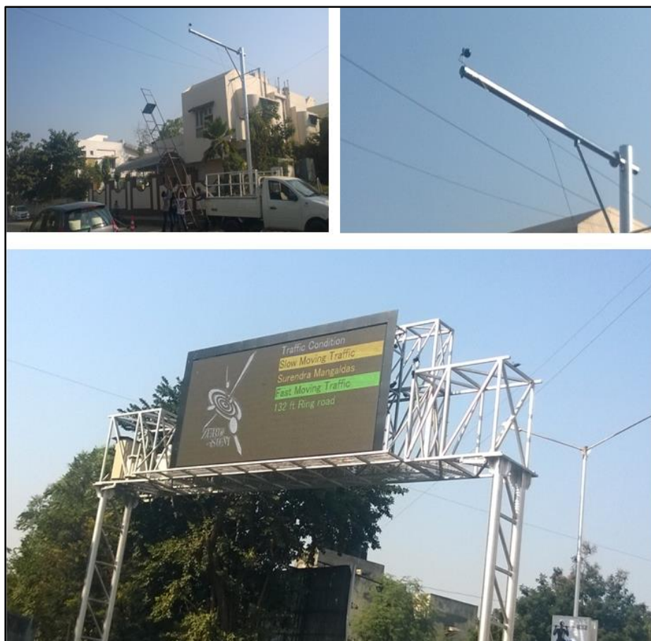
Figure 3-4: View of VMS and Cameras Installed at Shivranjini, Ahmedabad
