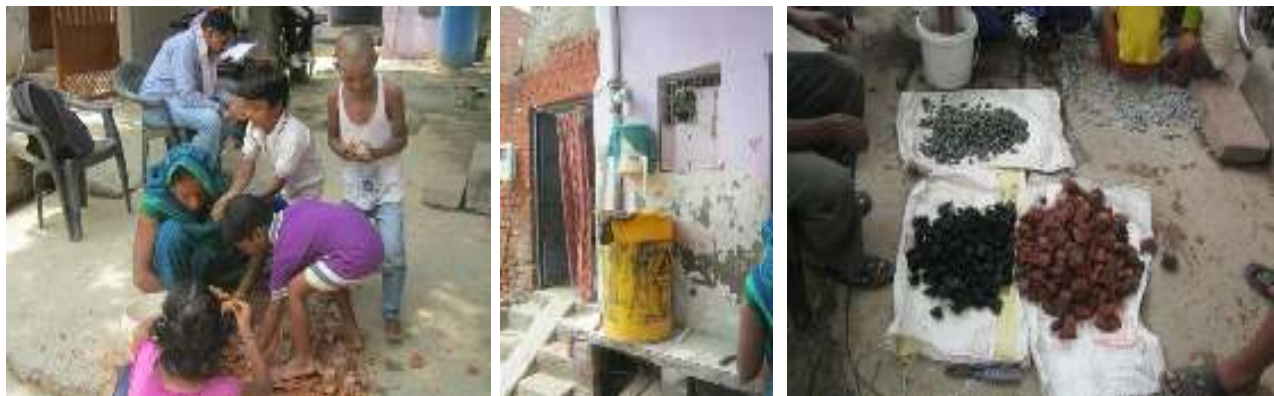
Figure 2: Household Retrofitted RWH System Being Installed by the Community
