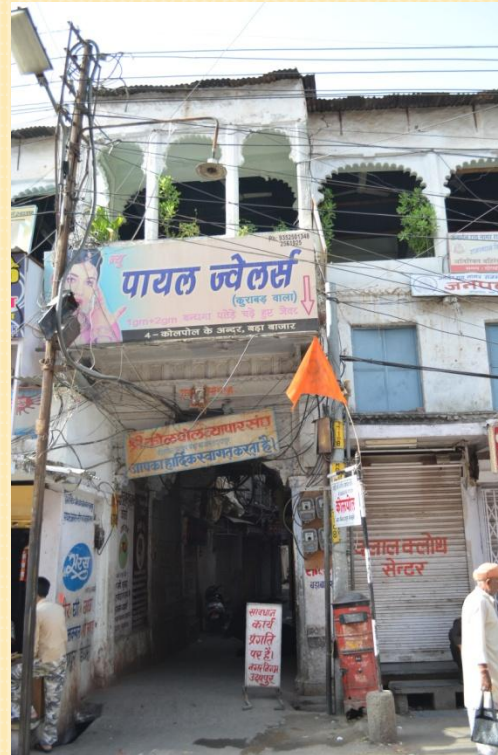
Disturbing building facade
