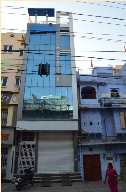
Disturbing building facade
