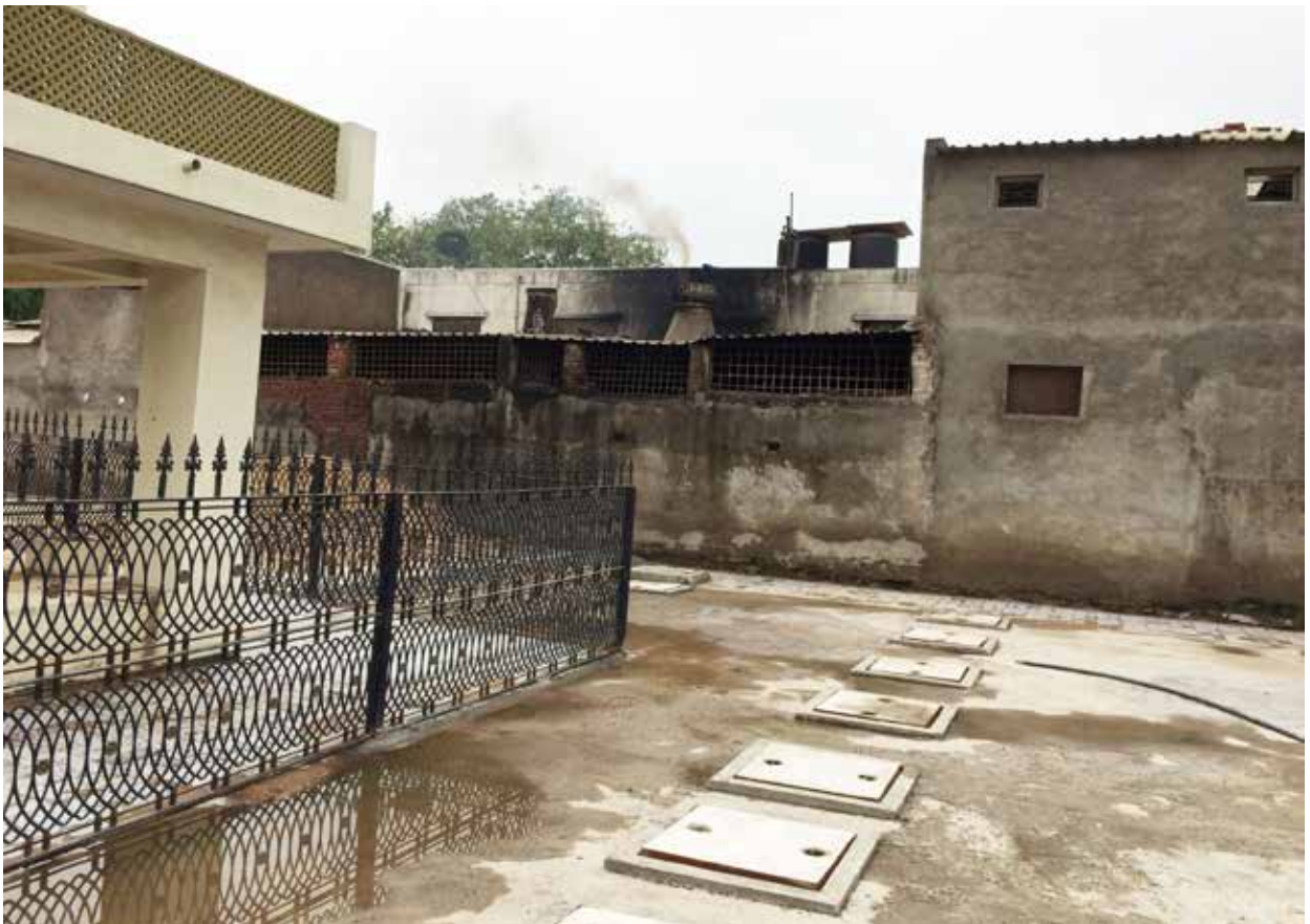
Decentralized Waste Water Treatment system in Rajkot India
