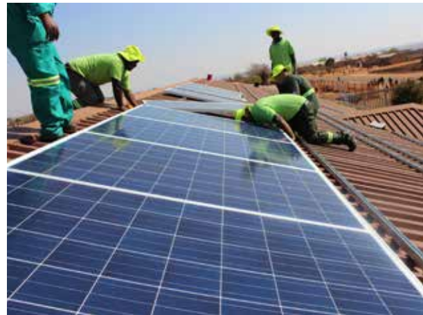
Solar Panel installation in South Africa Urban-LEDS
