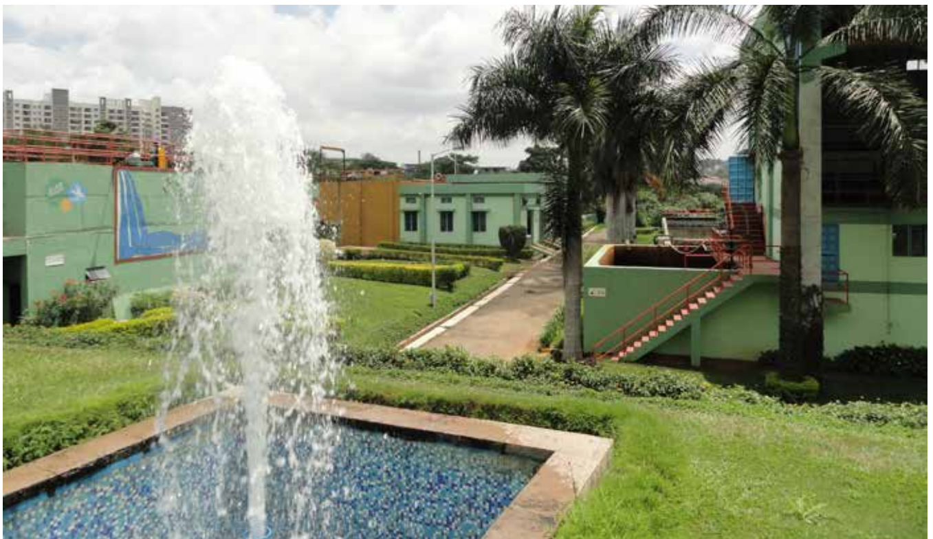
TREATED WASTE WATER FROM PLANT IS USED TO CATER THE DEMAND FOR NON-POTABLE USE
