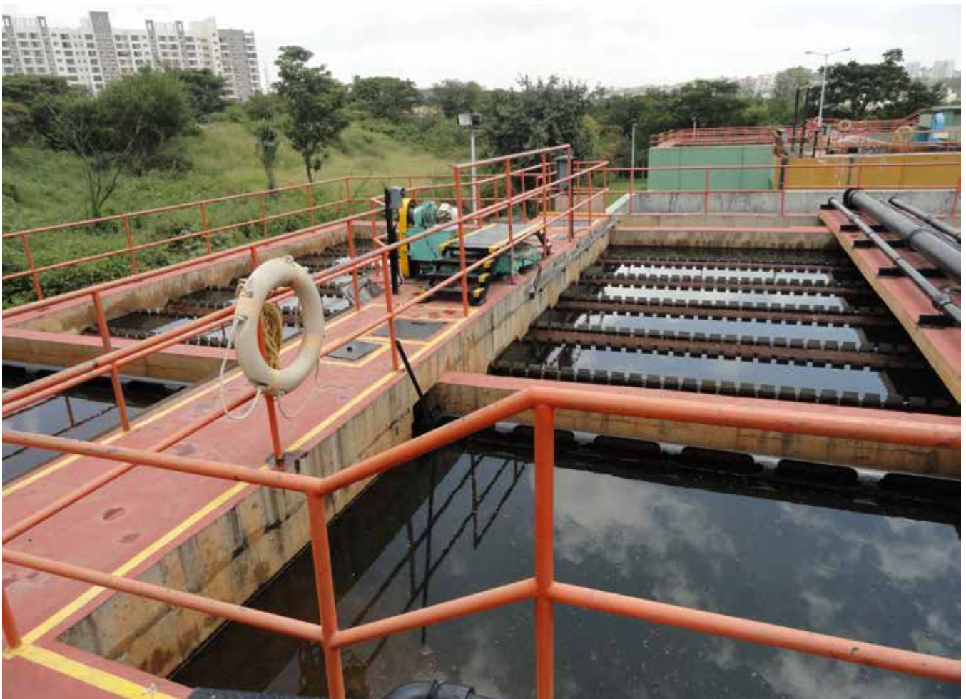
WASTE WATER TREATMENT PLANT
