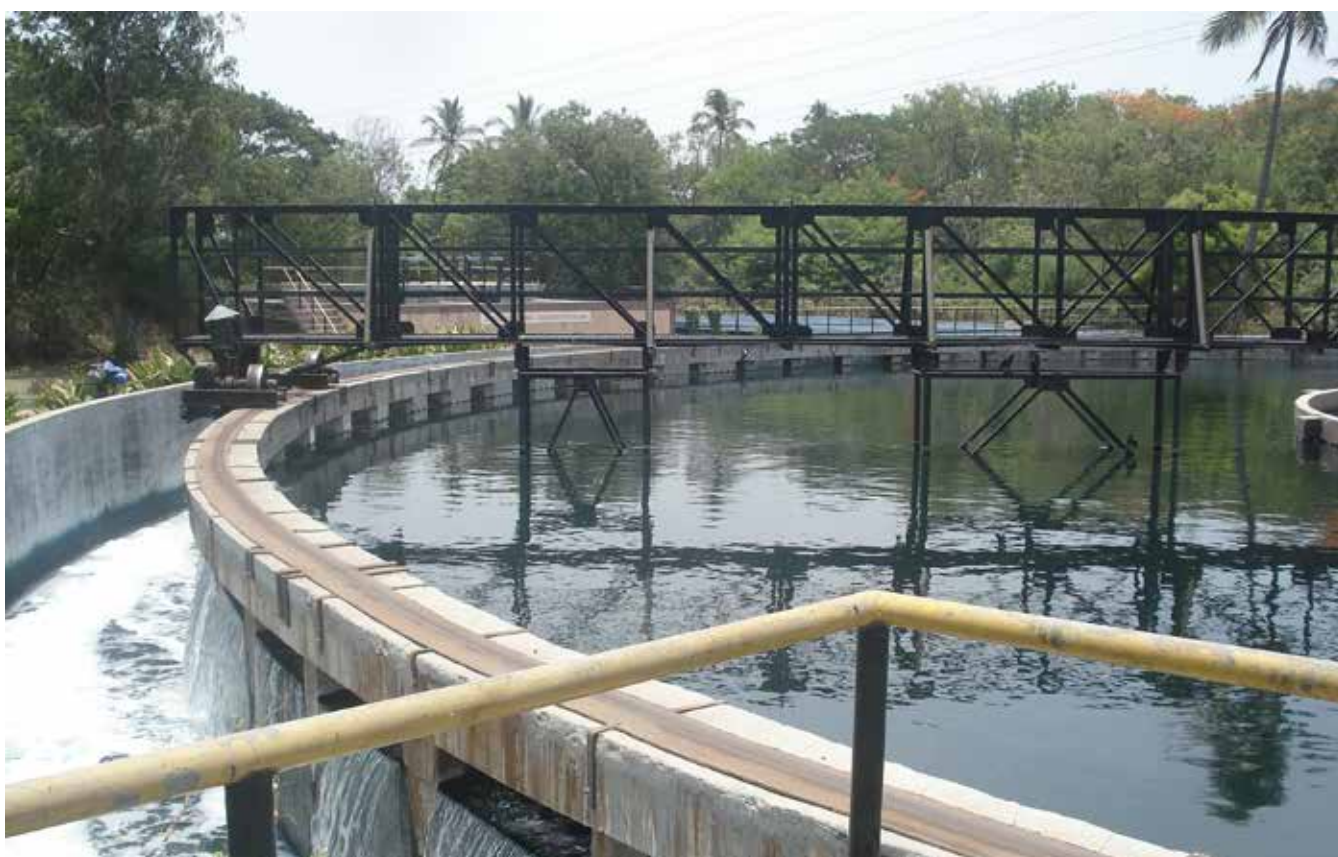
CLARIFLOCCULATOR, SEWAGE TREATMENT PLANT
