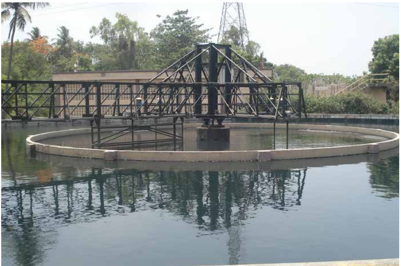
SEWAGE TREATMENT PLANT ,SURAT
