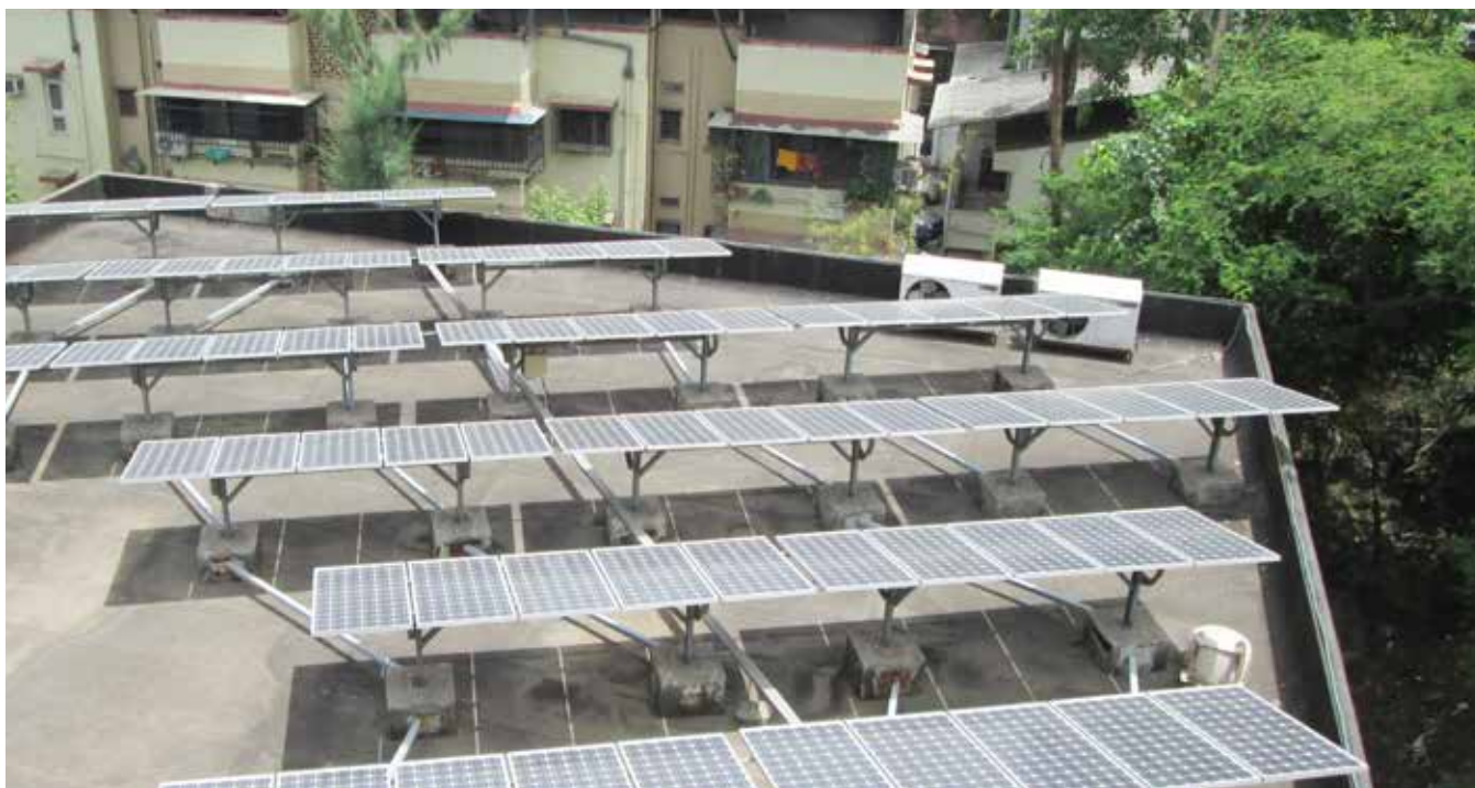
PHOTOVOLTAIC SYSTEM INSTALLED ON ROOFTOP OF THE BUILDING, THANE
