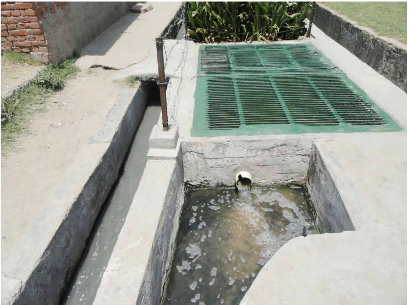
DEWATS IS TREATING BLACK WATER FROM UPSTREAM SETTLEMENT
