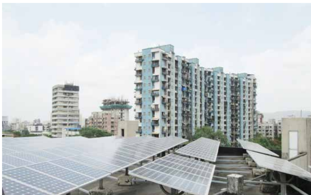
ROOFTOP PHOTOVOLTAIC POWER SYSTEM
