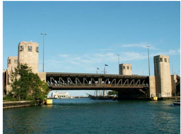
Figure 6. Lakeshore Drive Bridge, Chicago, 1937
