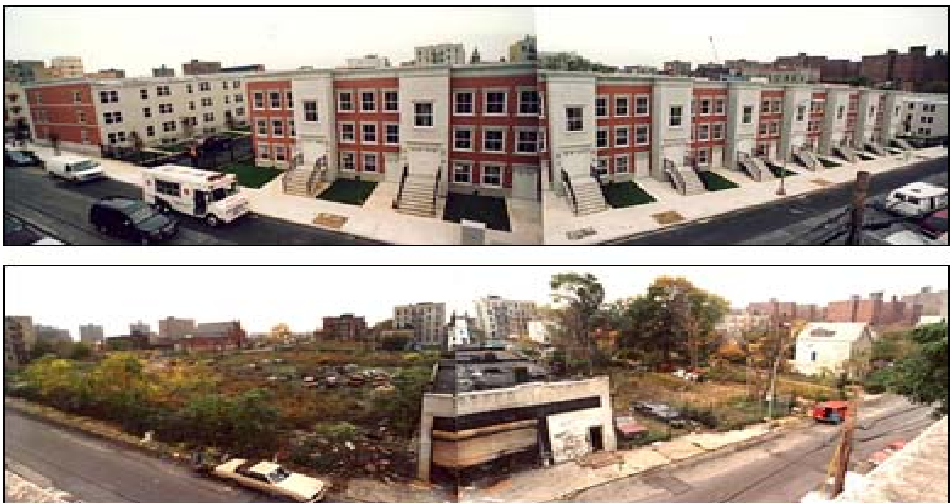
Figure 1. South Bronx after fire (bottom) and now (top)
