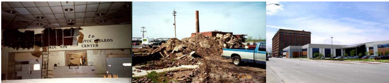
Figure 16. Butler World Headquarters construction. Kansas City, Missouri.
