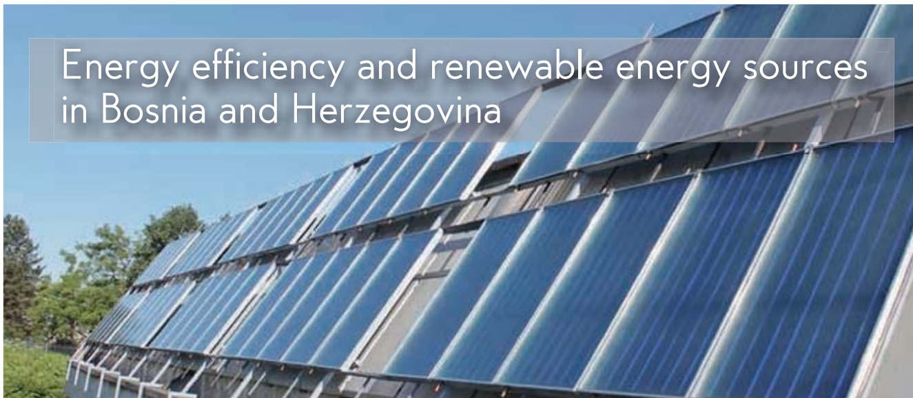
Thermal solar collectors at Sports and Culture Centre in Tuzla, Bosnia and Herzegovina
