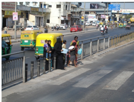
Picture 13: A pedestrian crossings that does not have a refuge area between the mixed traffic lanes and the BRT lane can be dangerous, if there are no pedestrian signals.
