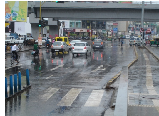
Picture 15: Here, the right turning traffic is allowed to merge with the BRT lane. This can be a safe solution, if this merging movement is signalised.
