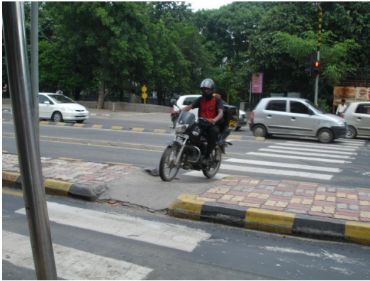
Picture 5: In the context of poor traffic discipline and enforcement in most Indian cities, road design should, as far as possible, dictate user behaviour. For example, provisions should be made to discourage or make it impossible for motorists to illegally use a pedestrian crossing to make a turn.
