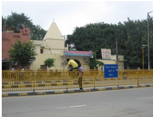
Picture 9: If adequate opportunities are not provided for pedestrians to cross the road, then they may resort to jumping the guardrail. Signage, as seen in the picture, does not serve the purpose.
