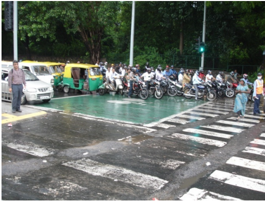
Picture 17: The green box marked on the road is meant exclusively for NMT, and the motor-vehicle stop line is advanced to just before the box. However, as is evident, given the poor level of traffic awareness and discipline, most motor-vehicles do not respect this design feature.
