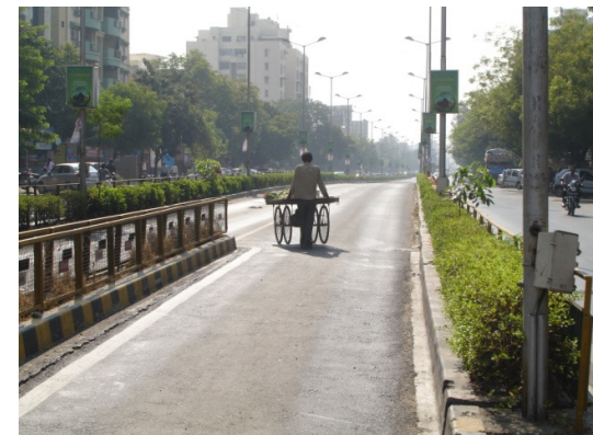
Picture 10: Since the gap between the bollards at the pedestrian crossing is not wide enough, the street vendor is forced to enter the BRT lane from the intersection, and then make a dangerous detour around the median, in order to cross the road.
