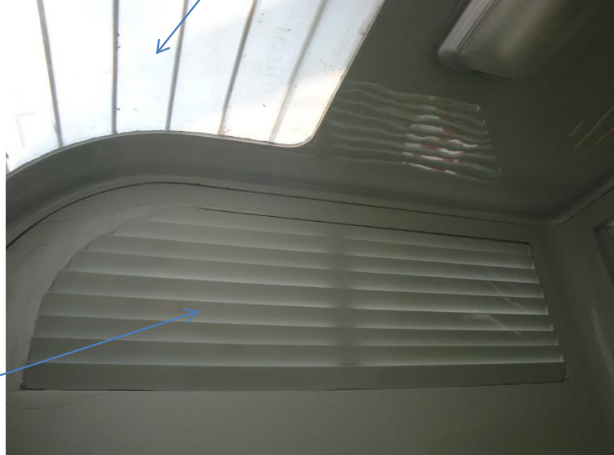
Natural air ventilation with provision of abundant Louvre arrangement
