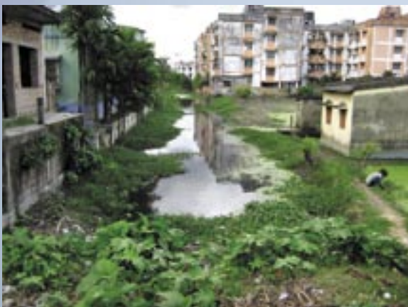
Drain carrying wastes to the lake
