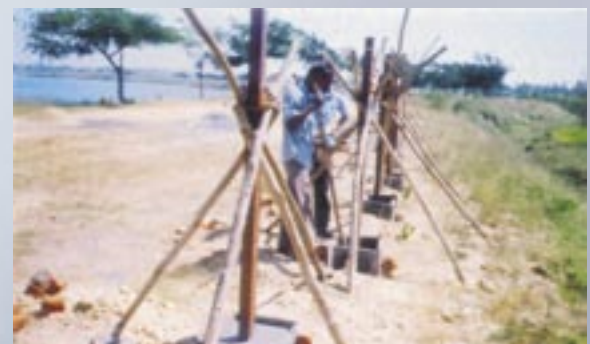
Work on Kundawada lake in progress
