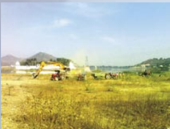
Desiltation of lake bed in progress
