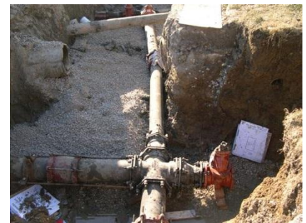
Photo: Inside a water main trench.
