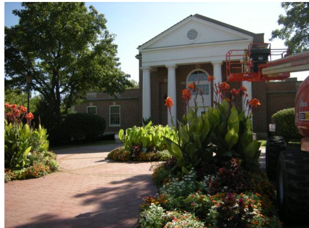
Photo: The western façade of City Hall was given a facelift in 2011, with lead abatement, column repair, and a paint job.
