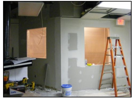
Photo: The new service windows at City Hall under construction, Summer 2010.
