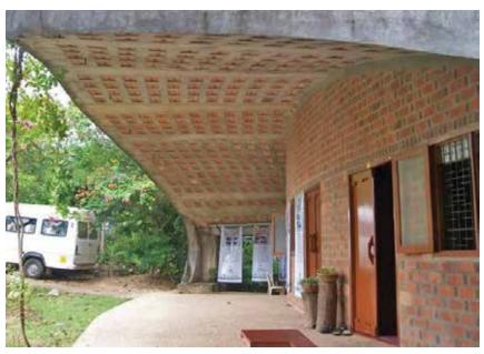
Picture showing a building at Laurie Baker Center, Trivandrum. Roof constructed using filler slab technique.
