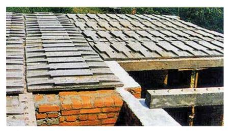
Roofing detail- Laying of precast RCC planks over RCC joists
