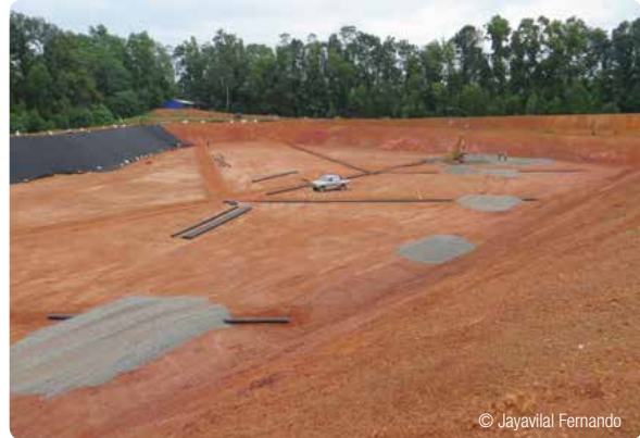
Sanitary landfill under construction
