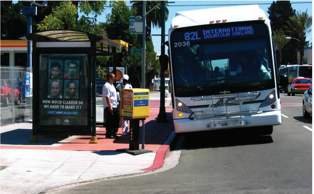
✓ This bus stop is located on a bulbout in the parking lane. Passengers can board directly from the curb rather than stepping into the street. Clear space for pedestrian movement is provided behind the bus stop.
