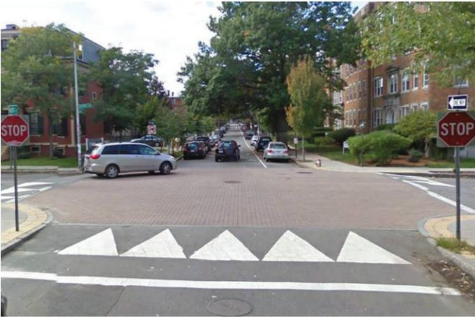
✓ Preferred design. The entire intersection is raised to the level of the footpath, compelling motor vehicles to slow down. The material difference alerts vehicle users that they are entering a shared space.
