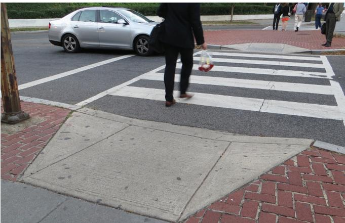
✓ Acceptable design for signalised intersections. If the crossing is at the level of the carriageway, each corner must be ramped. The width of the ramp should be at least 1.2 m, and the slope no steeper than 1:10 (IRC: 103-2012, 6.2.2, 6.5).
