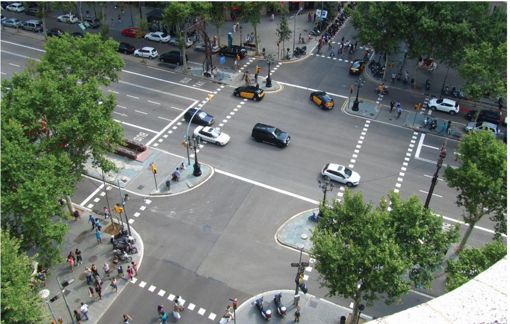
✓ Refuge islands can provide a safe place for pedestrians to wait for a green signal. They also reduce the crossing distance. The placement of refuge islands should reflect pedestrian desire lines.
