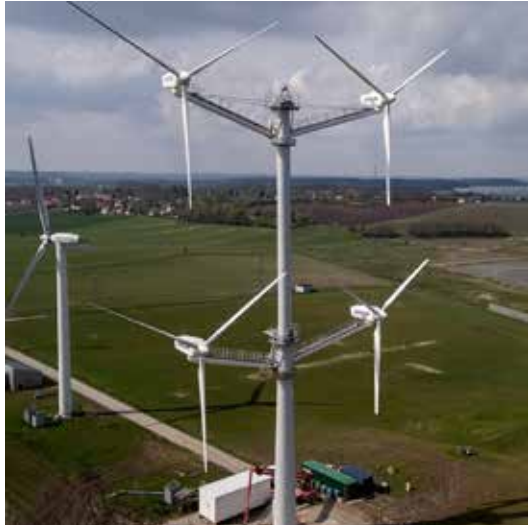
Figure 1.8: Wind Turbine with Multiple Rotors
