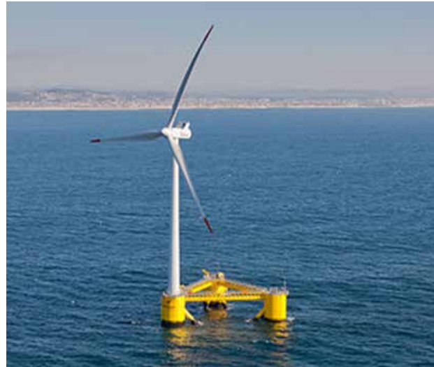
Figure 1.7: Floating Wind Turbine in Portugal
