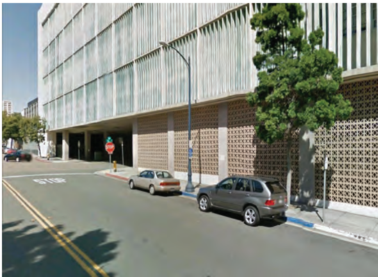
Figure 7.8: Blue zone parking area, San Diego, USA
