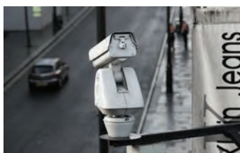
Figure 9.16: CCTV cameras at intersection
