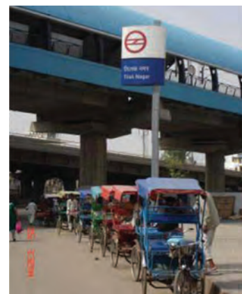
Figure 3.12: Cycle parking facility near public transport stand at Delhi metro station, India
