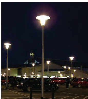
Figure 9.15: Pedestrian Street lights, USA
