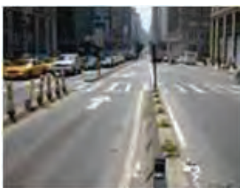
Figure 9.19: Manhattan Street - Before implementation
