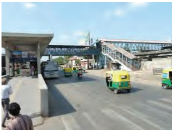
Figure 3.14: Interconnected BRT and Railway station through FOB, Ahmedabad
