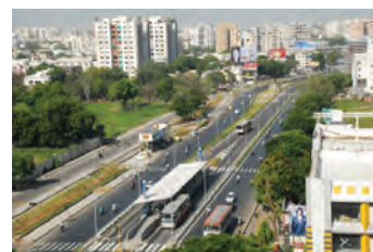
Figure 3.16: Bus rapid transit stops, Ahmedabad
