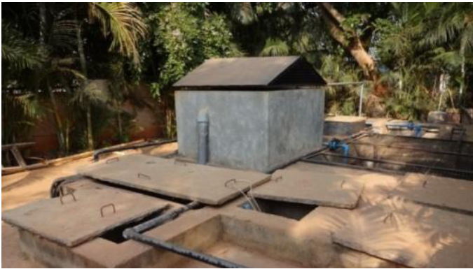
Picture 2: Sewerage treatment plant at ZED Collective Source: NIUA down.
