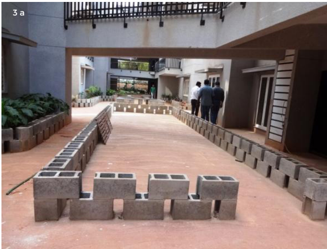
Picture 3: Reuse of construction left overs into landscaping Source: NIUA
