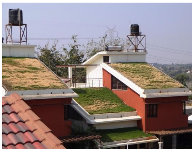
Picture 8: Green sloping roofs in villas Source: NIUA
