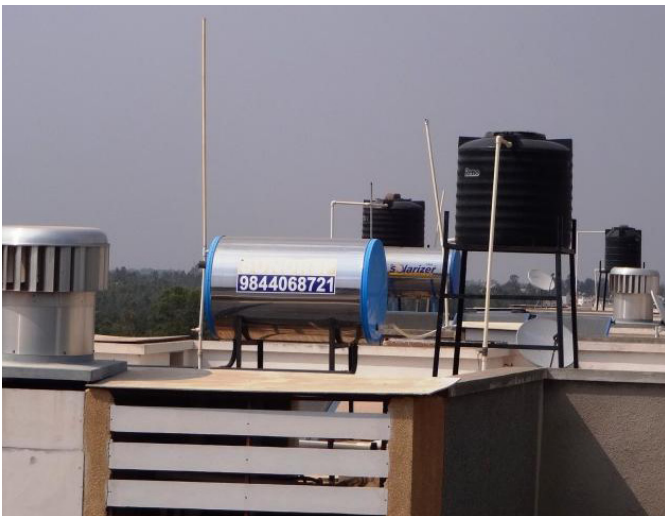
Picture 11: Exhaust of earth cooling system Source: NIUA
