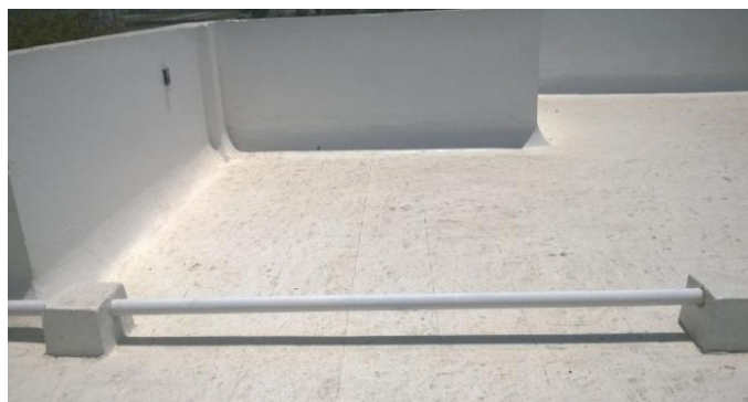
Picture 3: Reflective coating on roof in Niranjapur
