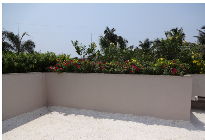
Picture 2: Some pilot sites where cool roof is being tested.
