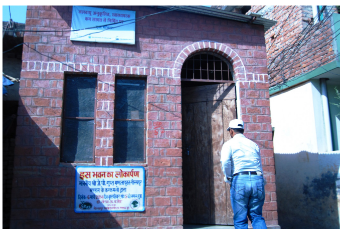
Picture 6: Demonstration unit of Climate resilient housing in Mahewa
