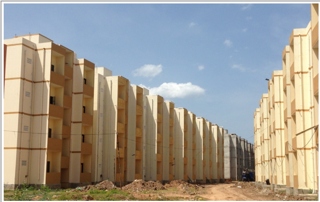
Photograph 4.2 - Multi-storey tenements that is under construction at Lambert Saravanan Nagar in Puducherry under JNNURM. It signifies the shift in policy focus on slum housing in the City.
