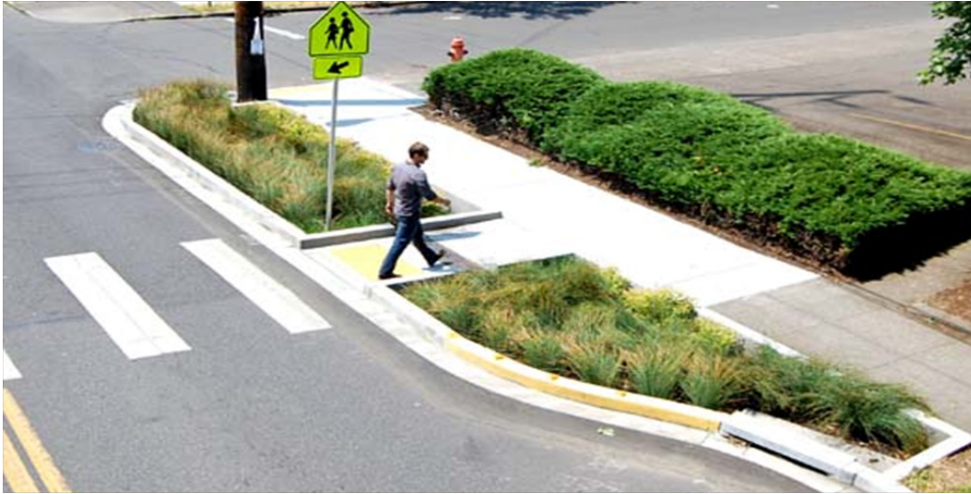
Figure 56: A bio-swale filtration system for ground water recharge integrated within street design
