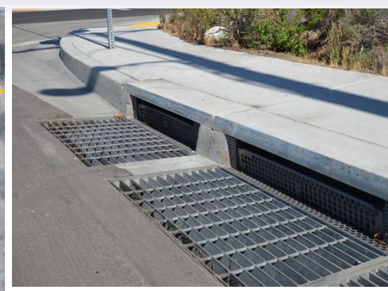
STORM WATER DRAIN
